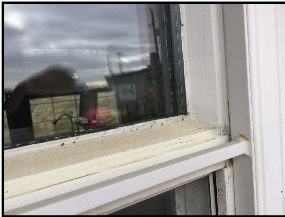
Photograph 3: Asbestos-Containing White Exterior Window Caulking.
