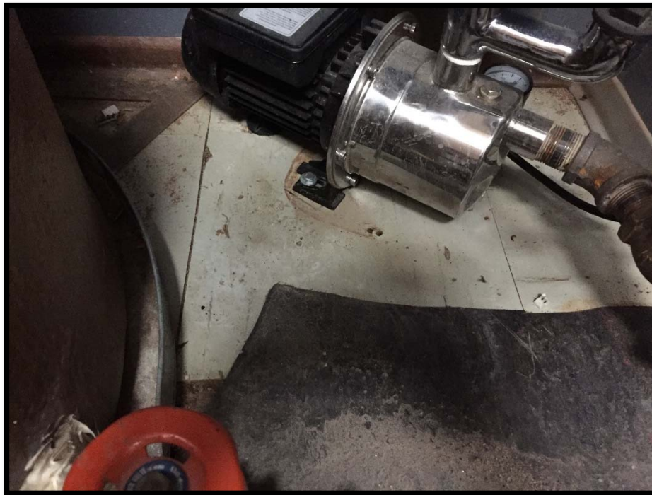
Photograph 2: Asbestos-Containing 12"x12" Off-White Floor Tile with Black Streaks.
