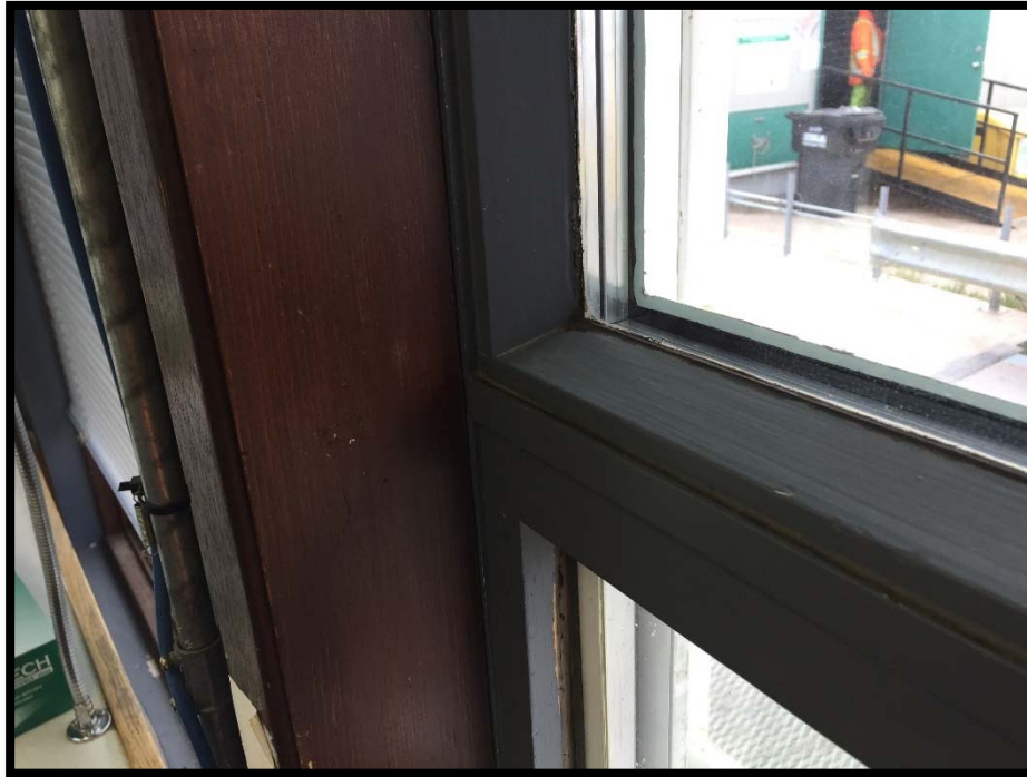
Photograph 1: Asbestos-Containing Black Interior Window Caulking.
