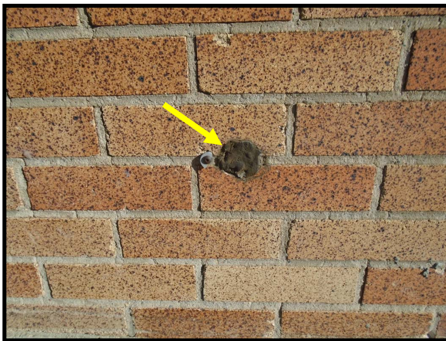
Photograph 1: Asbestos-Containing Grey Firestop Putty
