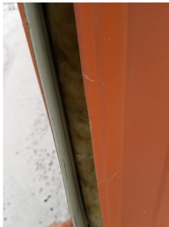
4) Fiberglass Exterior Wall Insulation (non-asbestos)
