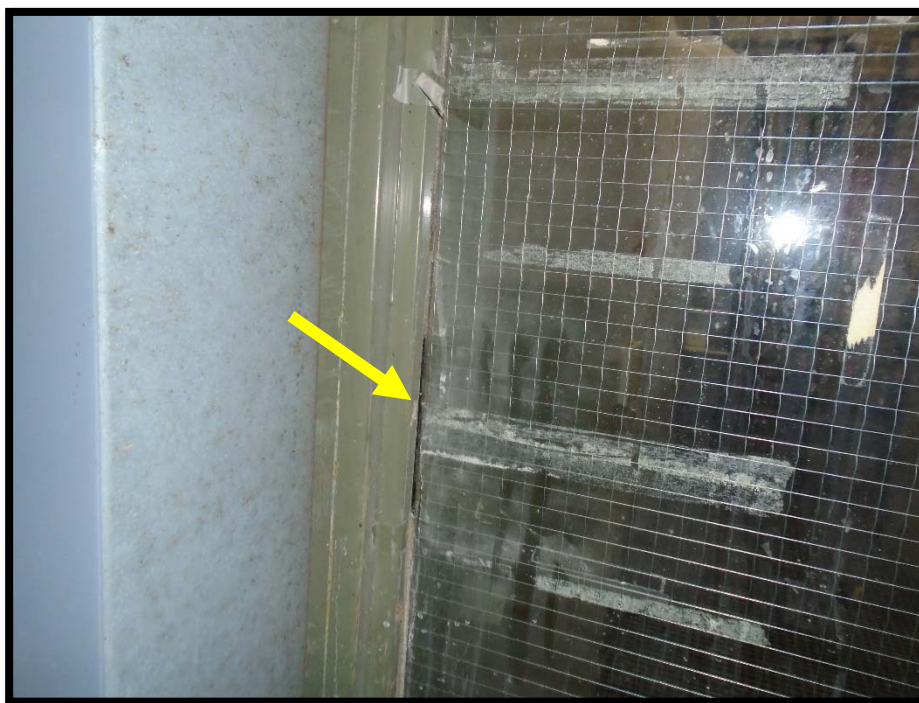
Photograph 1: Asbestos-Containing Black Window Glazing.
