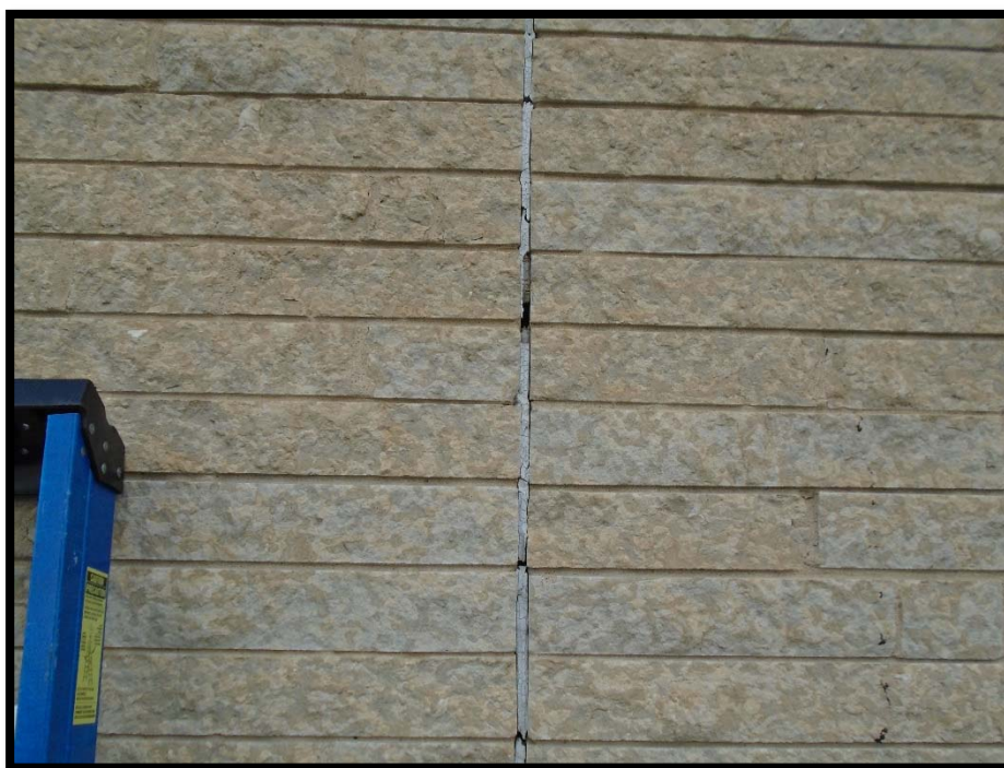
Photograph 2: Asbestos-Containing Grey Expansion Joint Caulking.
