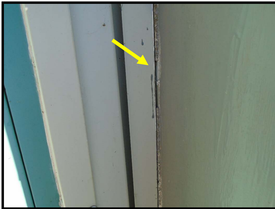
Photograph 1: Asbestos-Containing Grey Caulking
