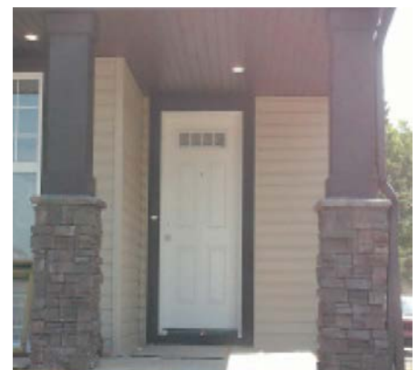
Wide-based columns with stone detailing. Preferred 10 inches x 10 inches columns or greater.
