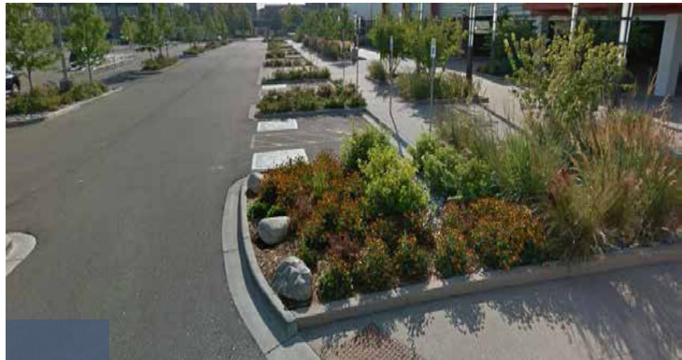
Curbed landscaped islands help buffer the presence of off-street parking spaces, while creating a more comfortable pedestrian environment.
