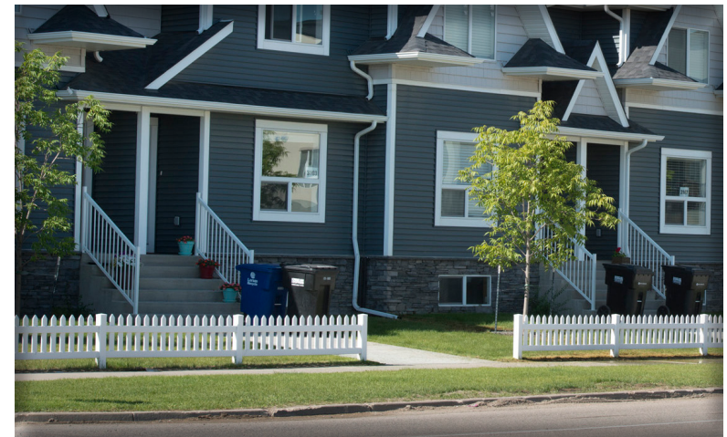
Above: Examples of acceptable front yard fencing
