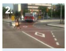
Geometric Priority Measures use queue jump lanes, and other roadway measures to provide buses with a time advantage at critical points along the corridor.
