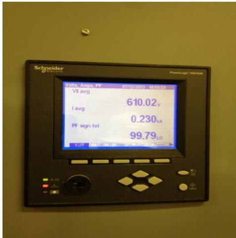
Monitoring equipment has been installed in 13 civic facilities to reduce utility costs and provide information that enables good management of facility equipment. The project involves installing a real-time data collection, reporting and analysis system that gathers utility consumption information from the facility. Industry research suggests that up to 5% utility cost savings can be achieved through utility monitoring.
