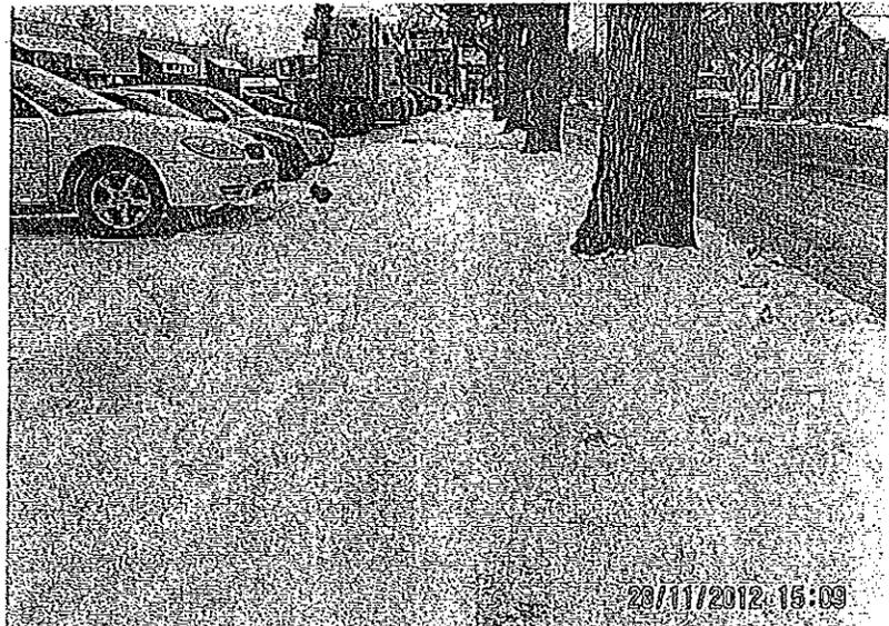
The adjacent picture is another example of a cleared compliant sidewalk. Again, there is clear evidence that there has been an attempt to clear a path with a width which is at least 1.2m. While there is some packed snow, the areas showing clear concrete is less than 3cm thick.
