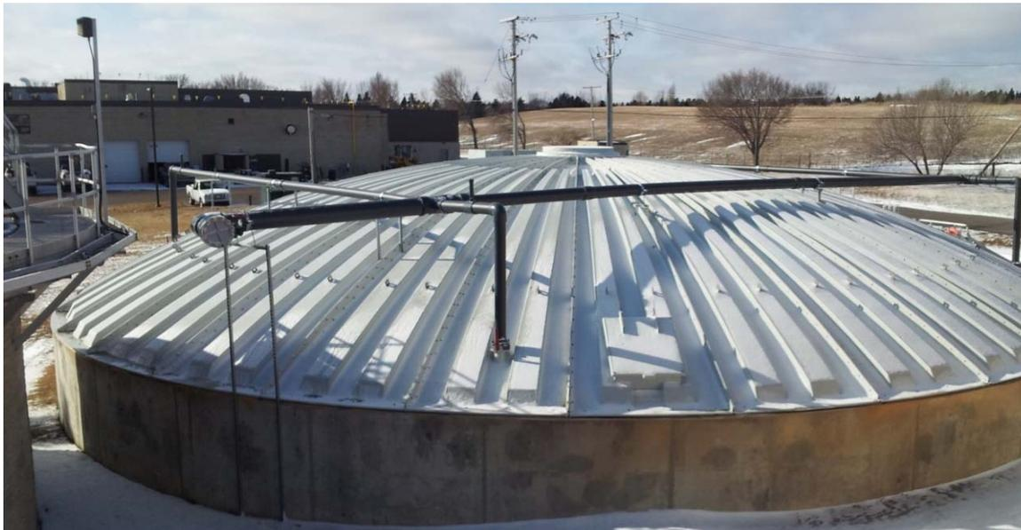
Waste Activated Sludge Stripping to Remove Internal Phosphorous (WASSTRIP) Tank
