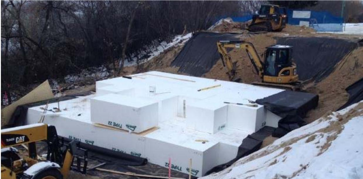
The above picture shows the expanded polystyrene fill used to stabilize the embankment.
