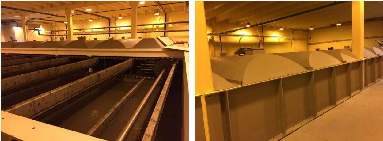
The above pictures show the WWTP Dissolved Air Flotation (DAF) tanks before and after covers have been added to reduce odour. The thickening process allows more solids to be removed from wastewater and contributes to the clarification process.
