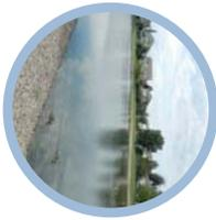
**WET PONDS** Storm water retention ponds that provide both retention and treatment of storm water runoff. A wet pond has a permanent pool of water.
