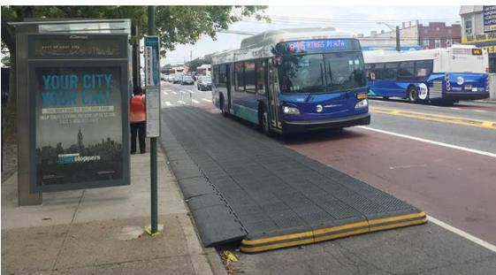
Transit platforms provide a raised landing area for passengers boarding and alighting transit. The platform eliminates grade changes for pedestrians, while providing a ramp on either end to accommodate cyclists passing over the platform. Shown is a temporary transit platform.
