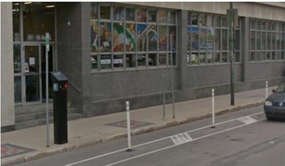
The white delineator posts would be used primarily at conflict points to provide guidance for motorist turning movements and additional protection for cyclists.
