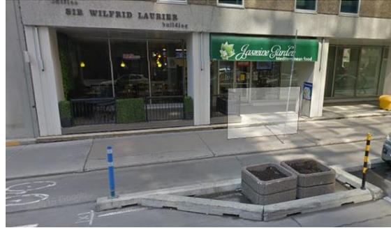
The addition of pre-cast curbing placed in the existing painted buffer area provides additional guidance for people parking, as well as additional protective barrier for people using the bike lane.
