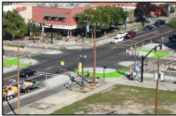
Protected intersection provide a high level of comfort and safety for bicyclists, especially at large intersections with multiple lanes and complex signal phasing. This design provides dedicated space for bicyclists extending into the intersections and as such can accommodate through, left-turn, and right-turn bicycle movements in a safe and low-stress manner.
