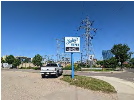
Electrical substation on Avenue C South
