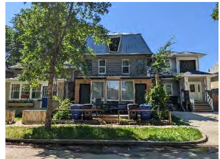
Multi-unit conversion of Riversdale character home
