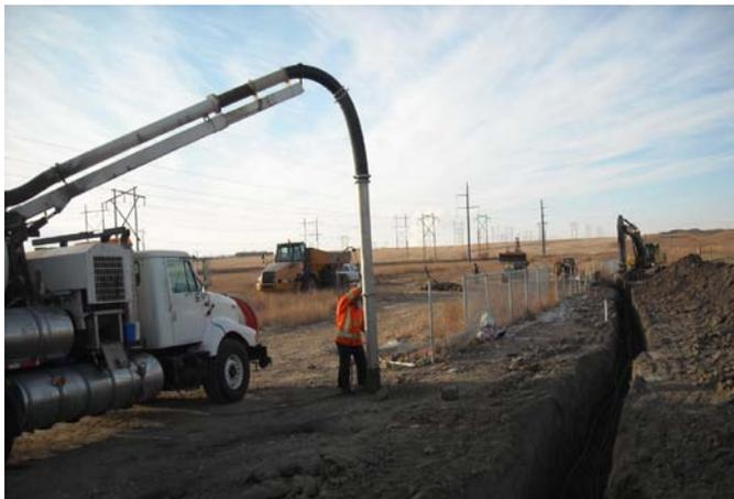
Installation of **leachate collection wells** to intercept groundwater that could come in contact with leachate from older unlined landfill cells.
