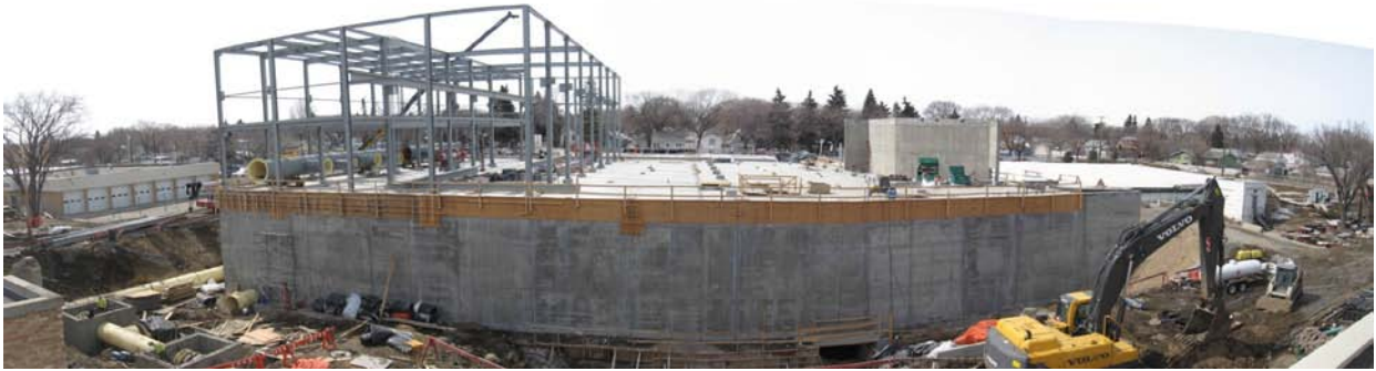
Aerial view of construction of Avenue H Reservoir Expansion
