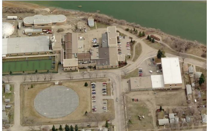
Aerial view of Water Treatment Plant and Meter Shop – Avenue H
