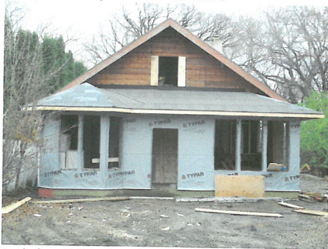
Back (west) Exterior - Nov. 2014
