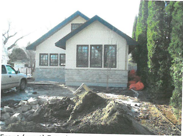
Front ( east) Exterior – March 2015
