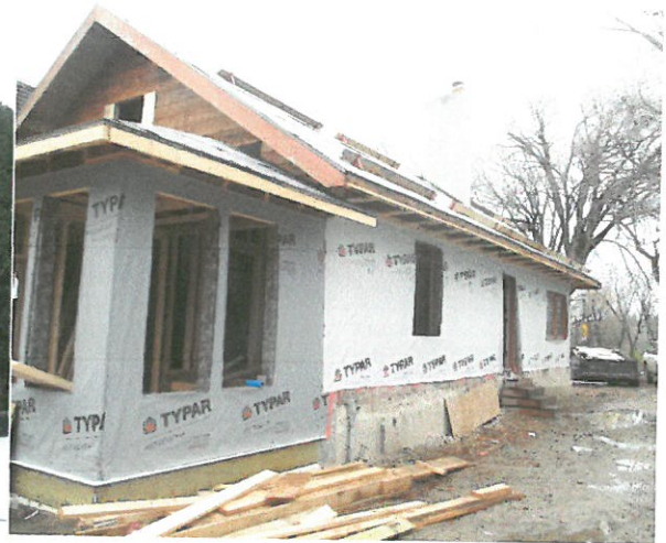
Side (south west) Exterior - Nov. 2014
