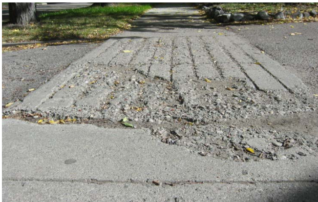
Figure 3: Spalling
