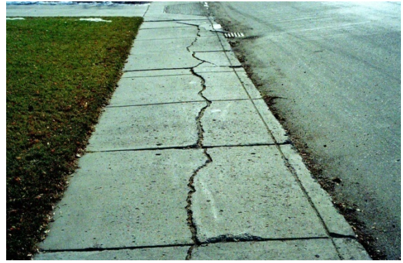
Figure 4: Longitudinal Cracking
