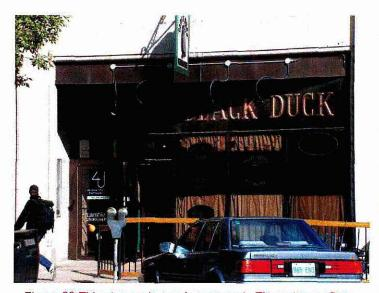
Figure 22 This store entrance is recessed. The entrance floor level is the same as the sidewalk, and the upper floor entrance blends with the other elements of the storefront. The use of coloured (pre-finished) aluminum doors blend with the storefront.
