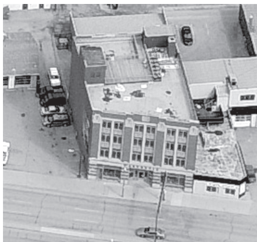
Fairbanks Morse Building, 14-23rd Street East.
