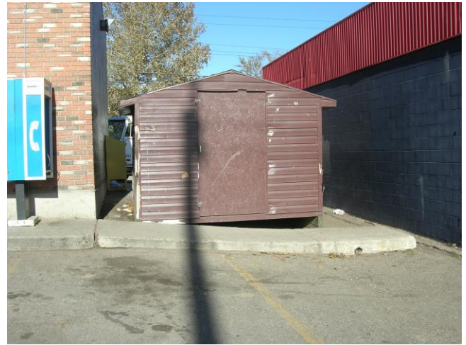
Entrapment area adjacent to convenience store
