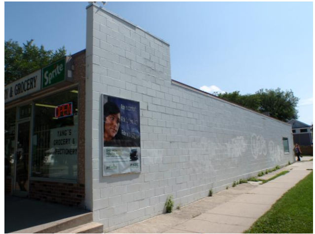
Evidence of graffiti vandalism removed from 29 th Street West convenience store wall
