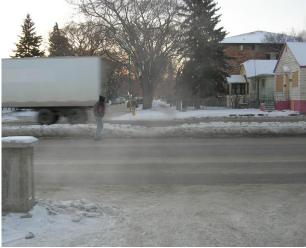
Pedestrian Crossing with Curb Cuts at the intersection of 22 nd Street West and Avenue K North
