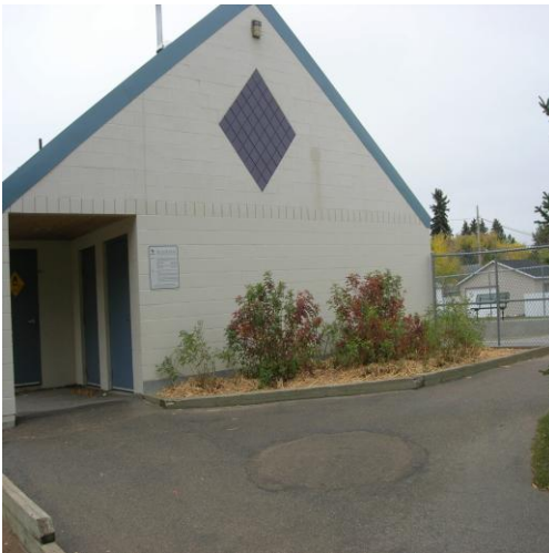
Westmount Paddling Pool and Recreation Unit Building
