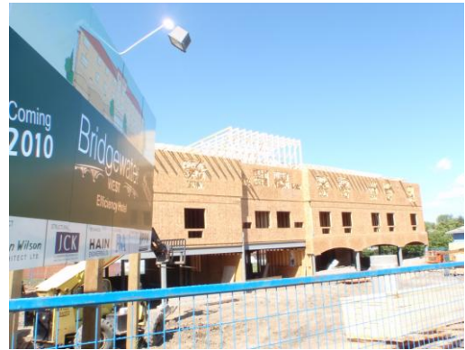
Bridgewater Hotel on 22 nd Street during construction
