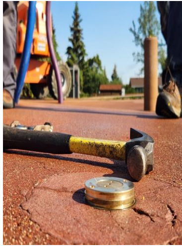
Improper Fit of Misting Nozzle
