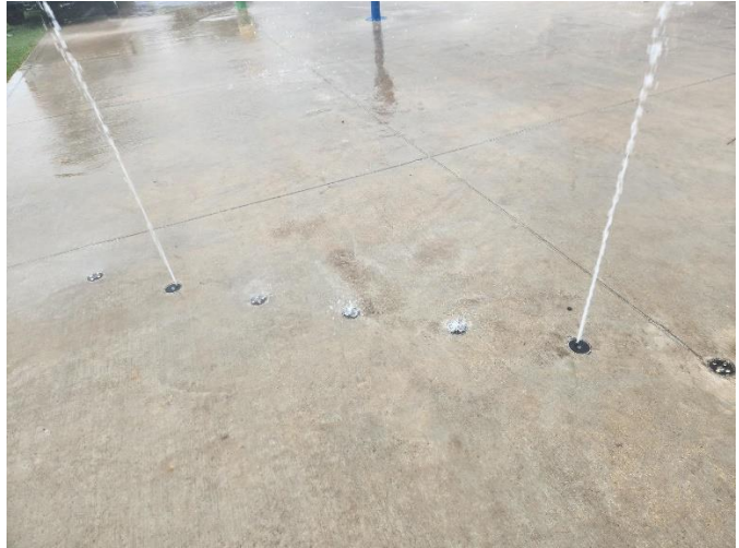
Misters didn't work at Stonebridge spray pad initially, but because of the nozzle design, after a couple of tries, we were able to overcome the water pressure limitation by increasing water volume.
