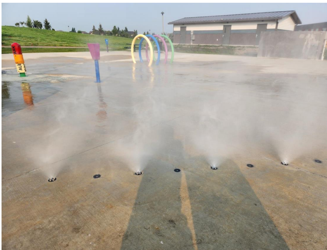
Misting Nozzles Installed at Stonebridge Spray Pad to Enhance User Experience
