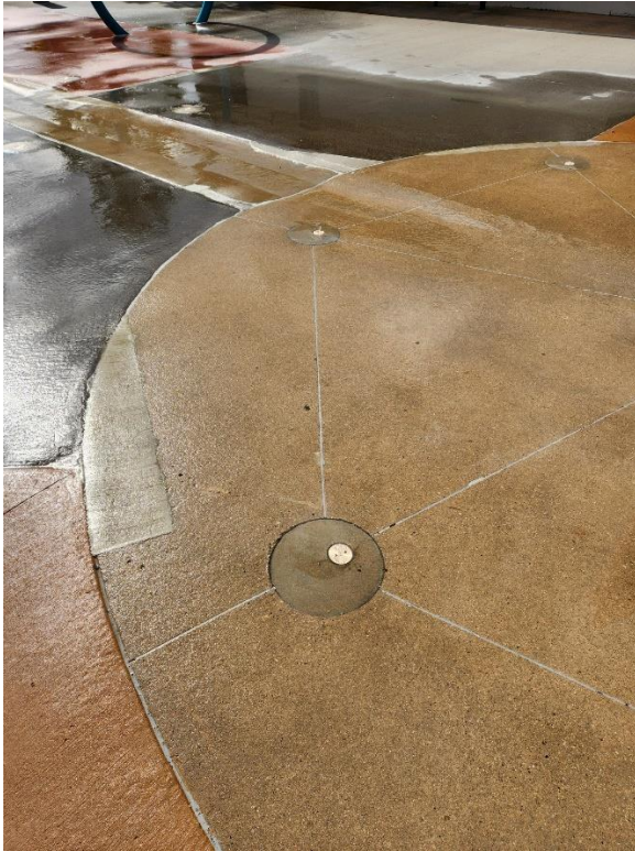
Misters didn't work at Briarwood Spray Pad because of issues with City water pressure. Nozzle design didn't allow water pressure limitation to be overcome by increasing water volume.
