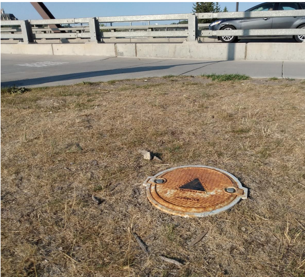
Flush-mounted monitoring well in a right-of-way
