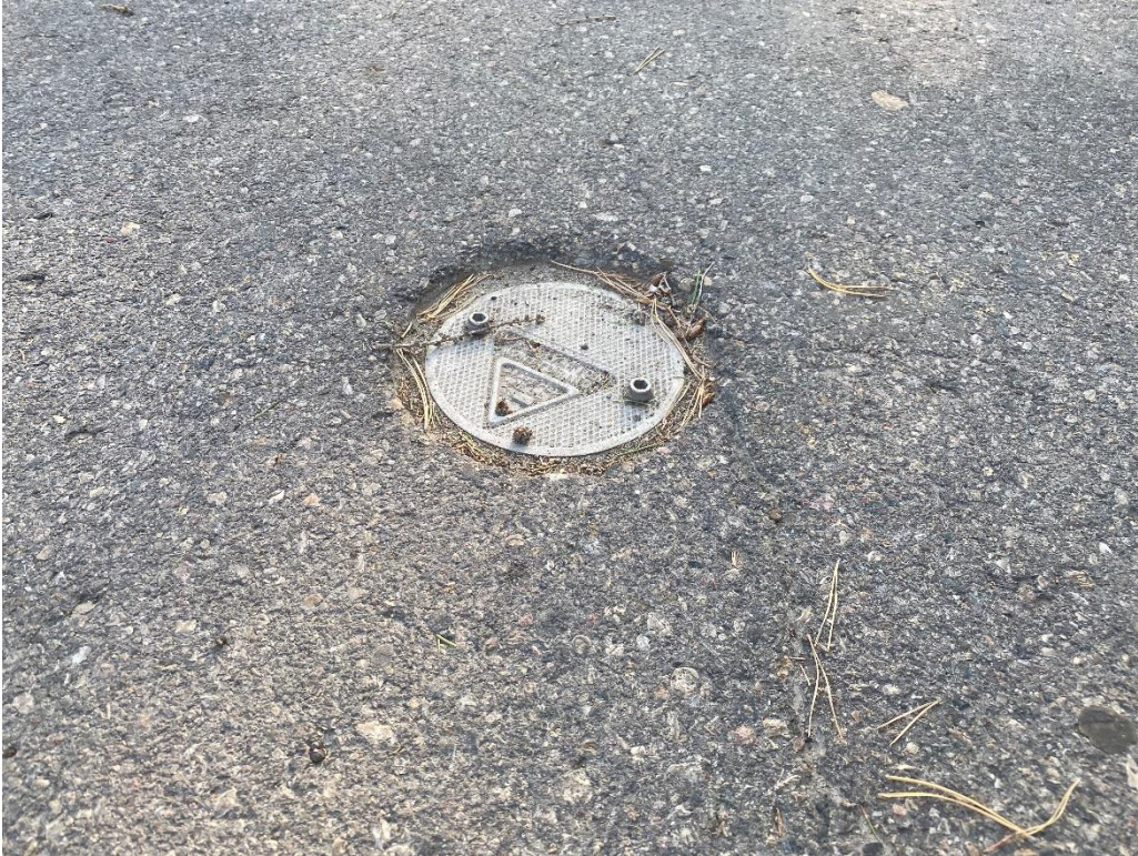
Flush-mounted monitoring well in a roadway
