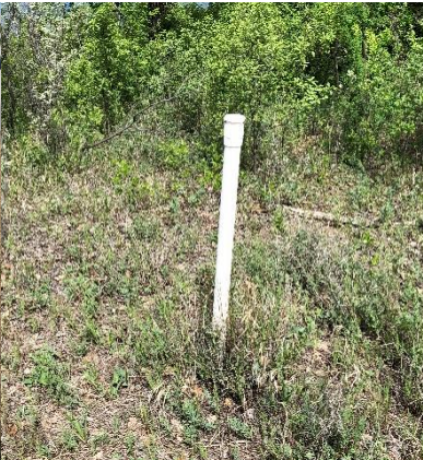
Fig. 3: Well with no protective casing
