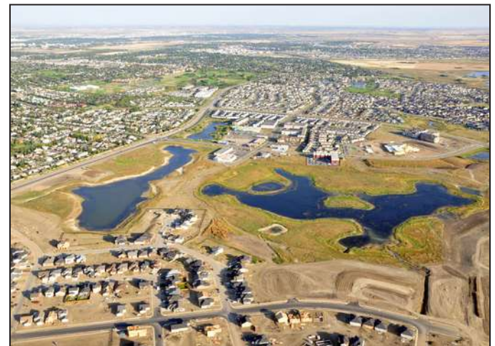
South-East Stormwater Management Area
