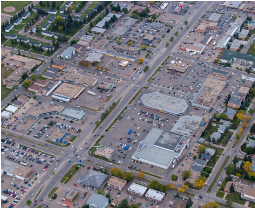
Figure 2: 8th Street East, a portion of the Red BRT Line Corridor
