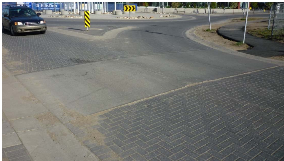
Exhibit 5-9: Textured Crosswalk using concrete in River Landing
