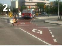
Geometric Priority Measures use queue jump lanes, and other roadway measures to provide buses with a time advantage at critical points along the corridor.
