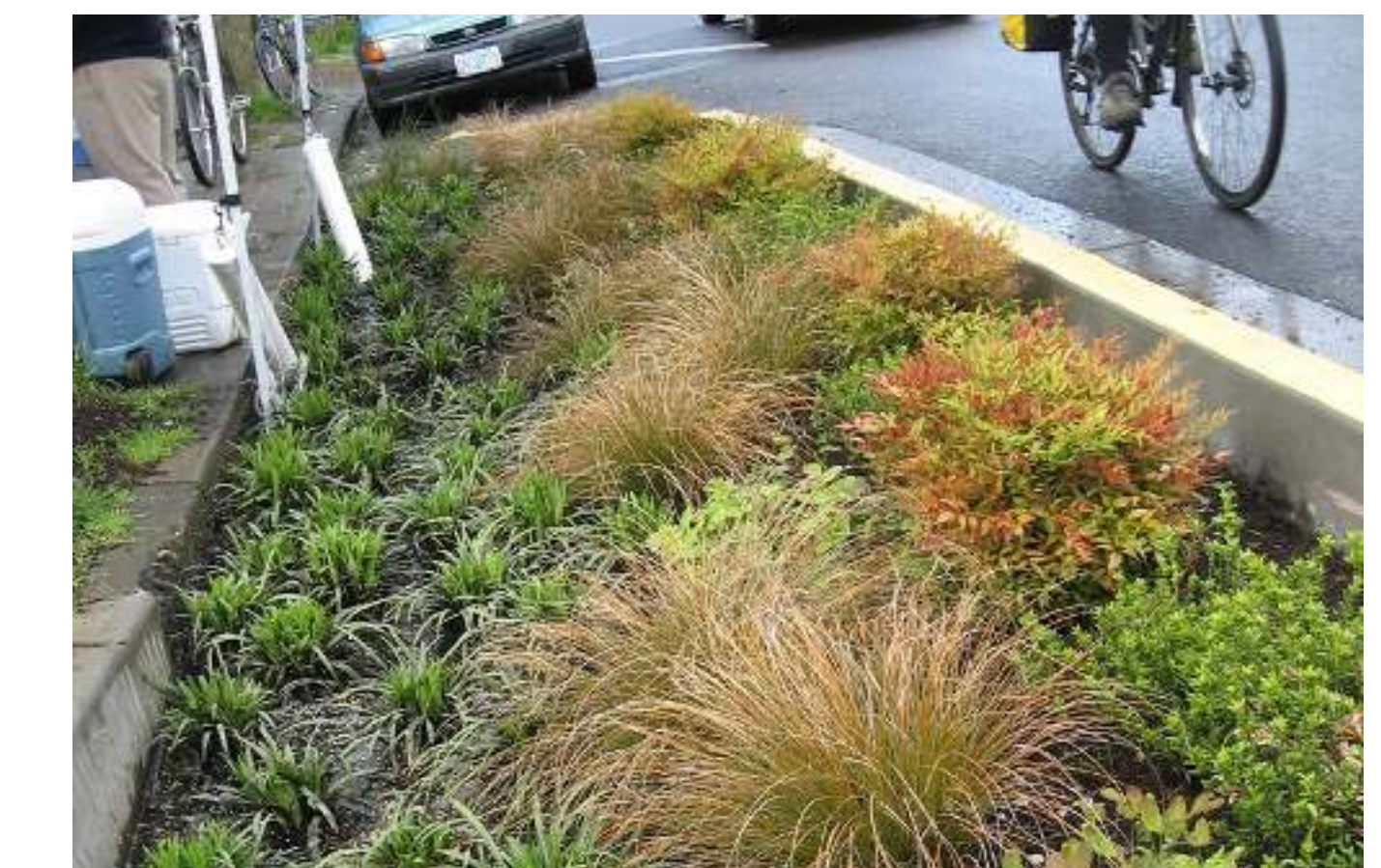
Bio-swales to filter stormwater run-off and facilitate local infiltration
