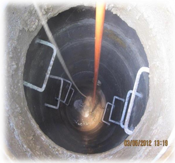
Closed Circuit Television Work
