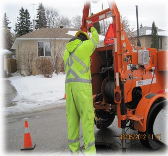
Closed Circuit Television Work
