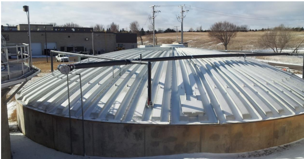
Waste Activated Sludge Stripping to Remove Internal Phosphorous (WASSTRIP) Tank with cover to reduce odour
