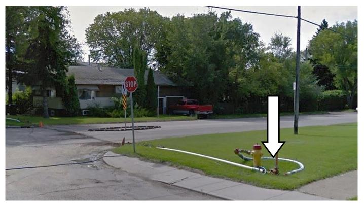
Typical set up. Hydrant adjacent to the construction limit will used as water resource during construction
