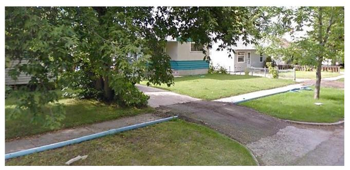
Pipe sections that will be connected together to form a temporary water main along the sidewalk. The contractor will make a ramp over the pipe at crossing with driveway or back-ally using appropriate materials
