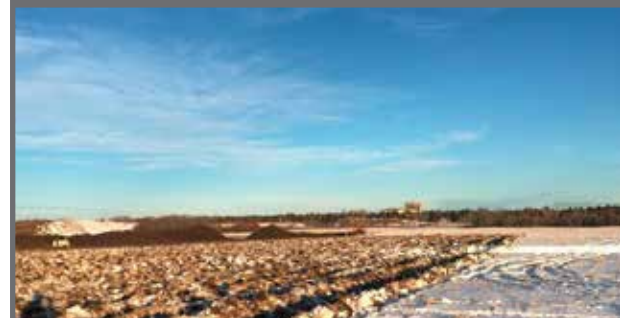
Removal of Topsoil on Site
