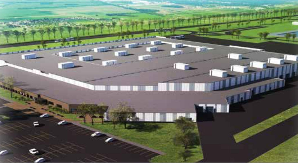
COC - Aerial View
