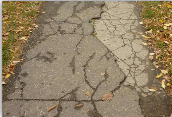
Poor Condition Asphalt Overlay Replacement
