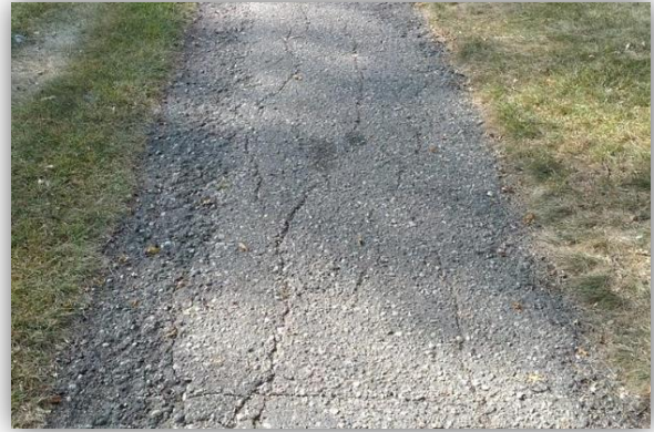
Fair Condition Asphalt Overlay Replacement or Overlay/Seal
