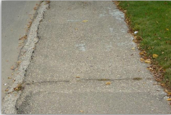
Good Condition Asphalt Overlay Curb Deteriorated - Replacement
