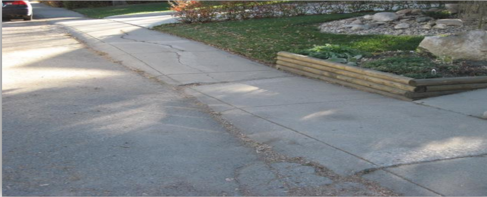
Utility Settlement – Mud Jack or Replacement
