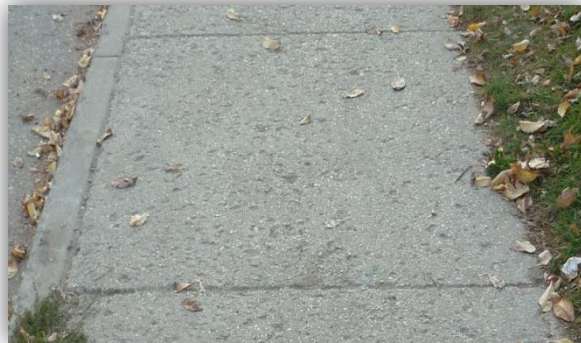
Light Severity – Silane Seal
