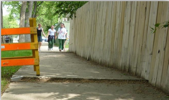
Repair – Grinding or Saw Cut
