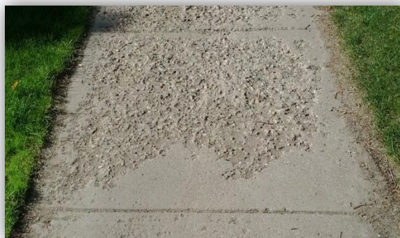
High Severity – Replacement
