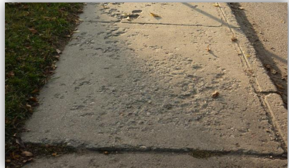
Medium Severity – Replacement
