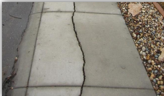
Repair - Crack Fill
