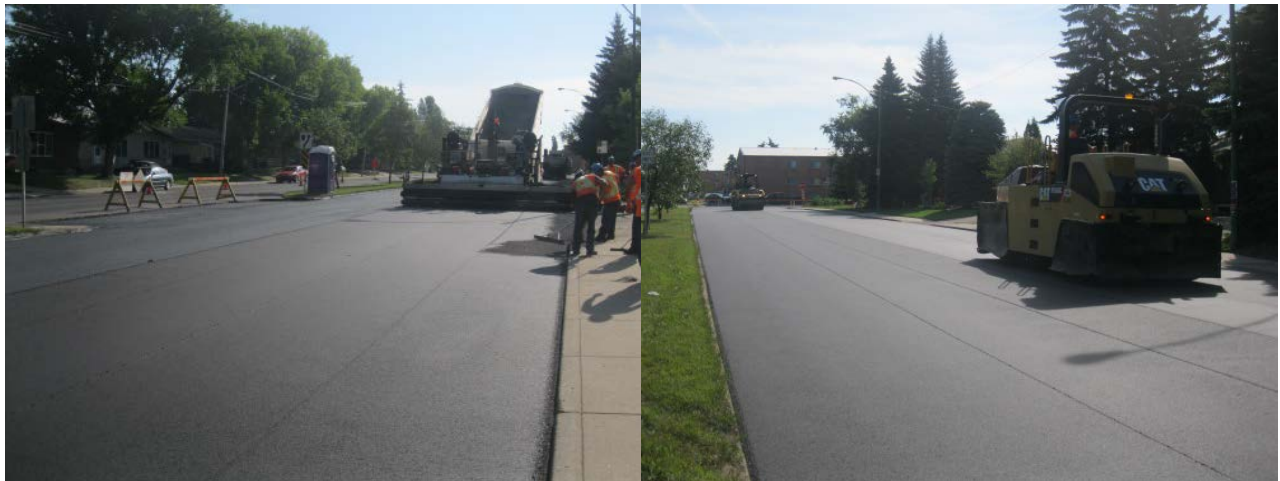
Typical Ultra Thin Overlay Project
