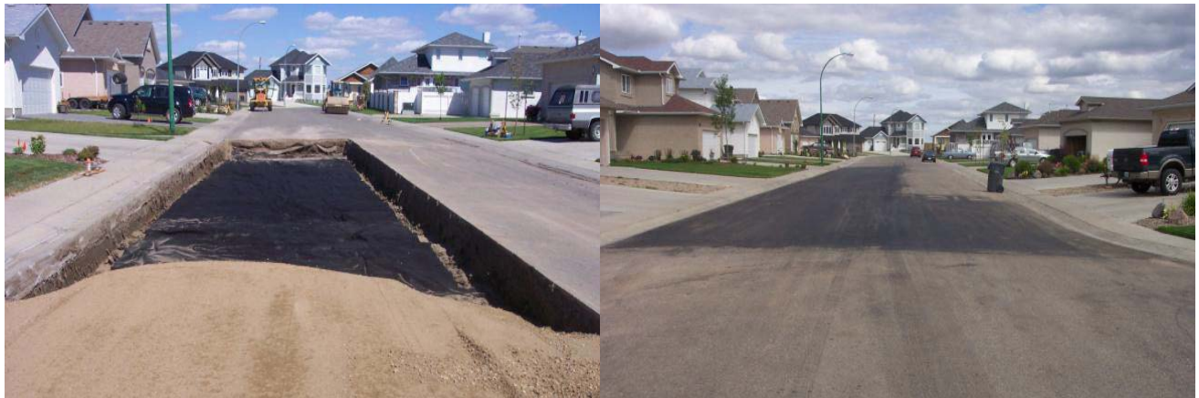
Typical Patching Project
