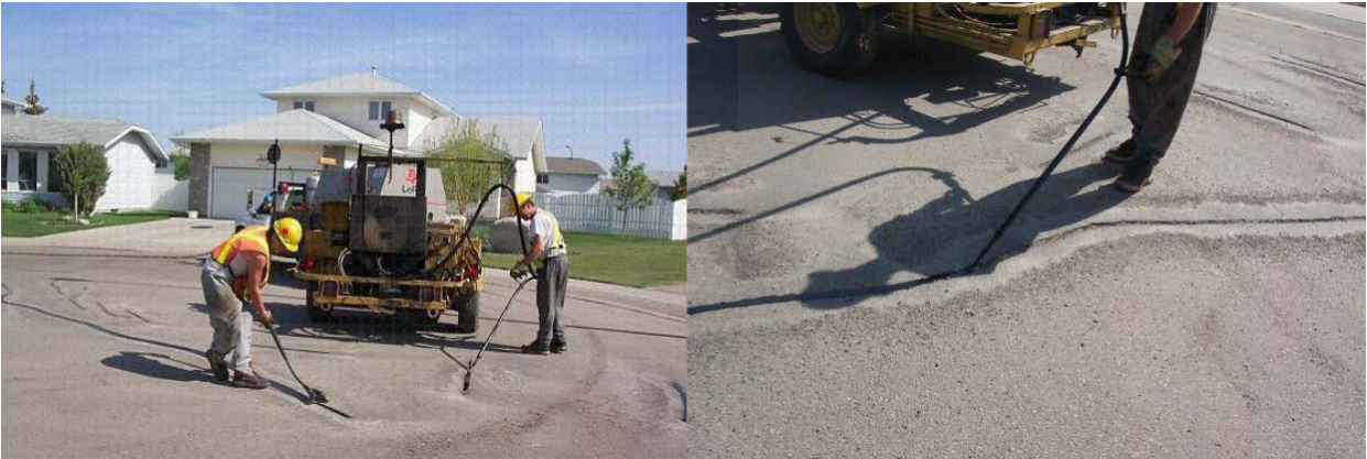
Typical Crack Filling Project
