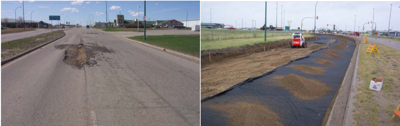
Typical Reconstruction Project
