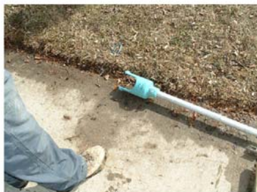
Curb Stop Spindle and Casing
