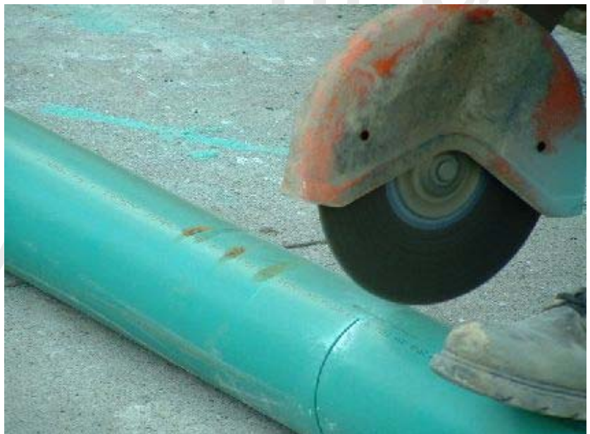
Figure 38 - Cutting Sewer Pipe
