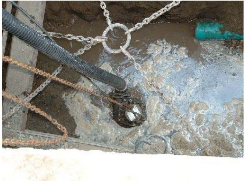
Figure 27 – Pump in Excavation.
