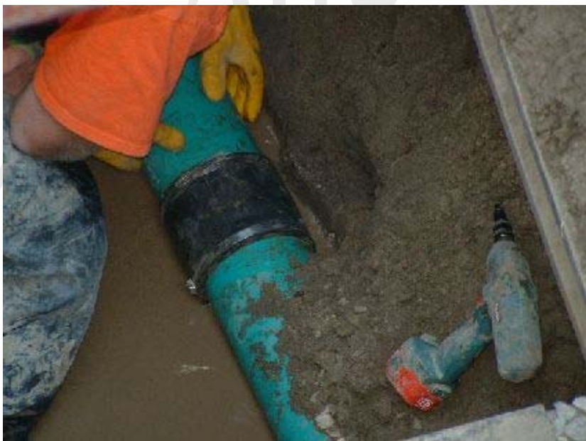
Figure 44 Aligning pipe
