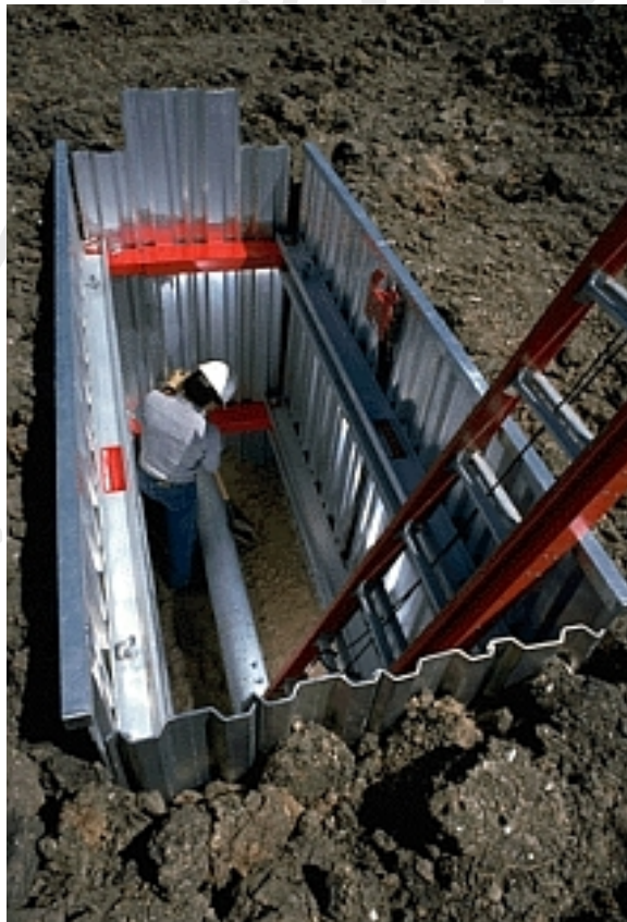
Figure 32 – Shoring with Endplates.
