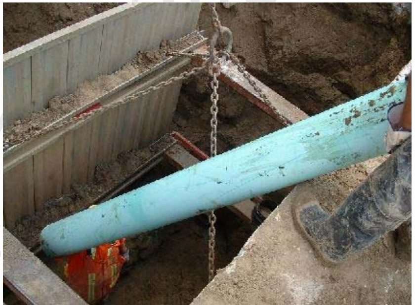
Figure 42 – Lowering Pipe
