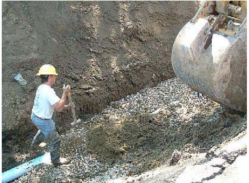
Figure 41 - Compacting bedding.
