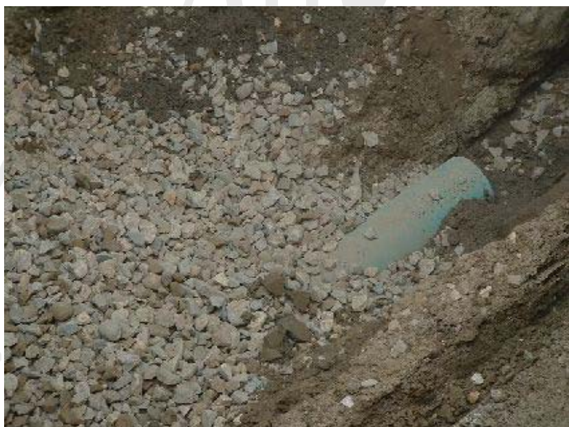
Figure 40 - New pipe over crushed rocks.
