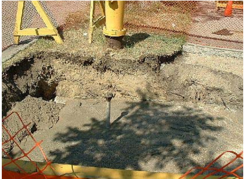
Figure 48 - Non-shrink backfill
