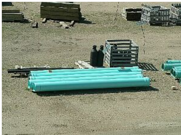
Figure 91 - PVC Sewer Pipes
