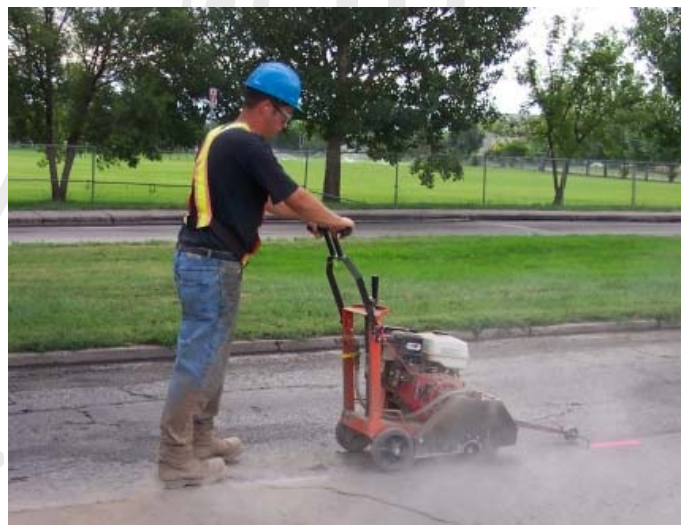
Figure 10 – Cutting Asphalt
