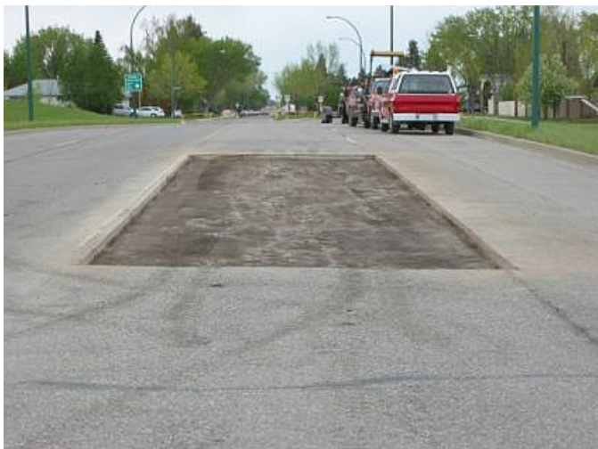
Figure 57 - Finished Backfill
