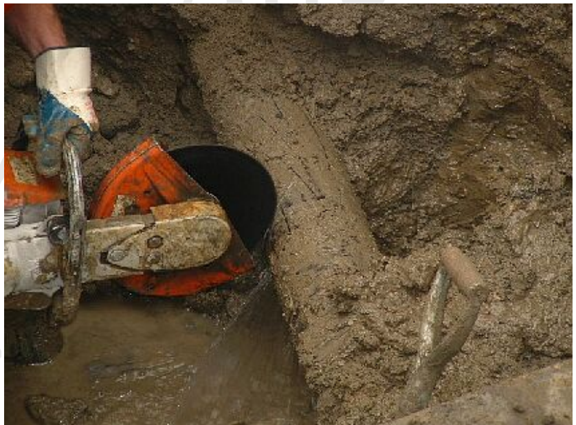
Figure 28 - Water Main Removal
