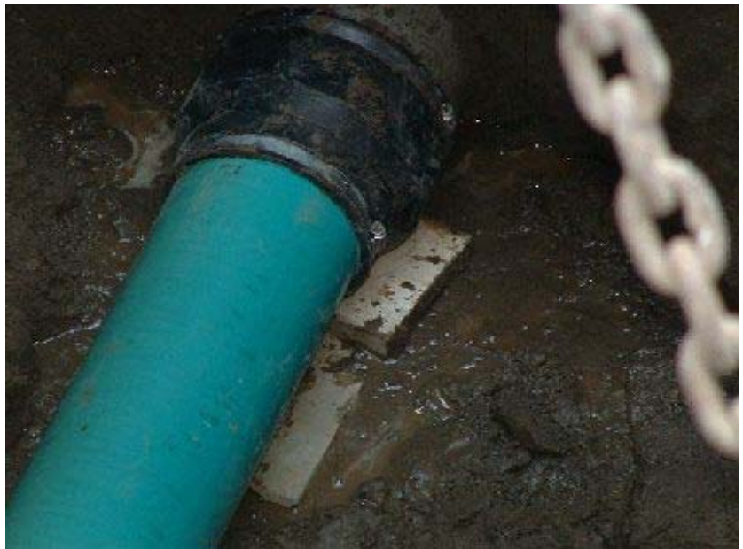
Figure 45 - Blocked Coupler
