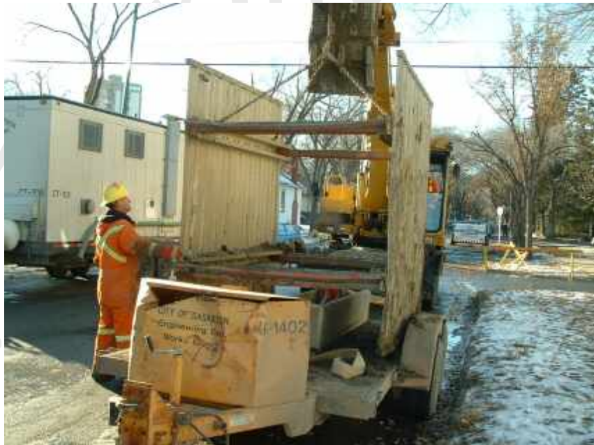
Figure 30 - Shoring being lifted off the trailer.
