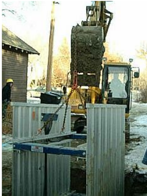
Figure 31 - Shoring Installation
