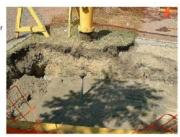
Non-shrink backfill shall be used beneath (concrete or paving stone), sidewalks or driveways. Leave non-shrink backfill a minimum of 300mm (12inch) below grade.
