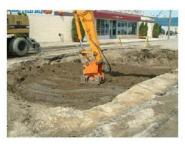
Hydraulic tamper is an attachment for the excavator. It is used to compact the soil.
