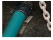
Block couplers so they will not offset during backfilling
