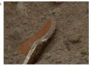
Cut pipe and roll out of bedding. Pipe may be removed later or broken into small pieces.
