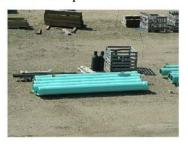
PVC (Poly Vinyl Chloride) pipe is the sewer main pipe used at the City of Saskatoon.
