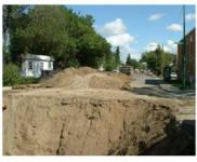
Material from the trench will be sorted into salvageable material (wet or dry) and non-salvageable material. If stockpiling of salvageable material on site is not a viable option a dumpsite will be used. The toe of the spoil piles must be a minimum of 1m (3Feet) from the edge of the excavation.
