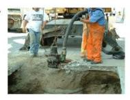
Lower a pump into the manhole upstream of the sewer repair. Connect and place the discharge hose in to the nearest manhole that will not interfere with the repair work.
