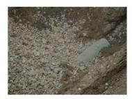
Proper preparation of bedding is critical. The Supervisor IV will approve the bedding before the pipe is installed.
