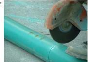
Cut the replacement sewer pipe with the quickie saw. Safety goggles and a facemask must be worn when using the quickie saw.
