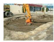
Hydraulic tamper (excavator attachment) cannot be used closer than 1m(3feet) directly above pipe or service. Use with 150mm (6inch) lifts.
