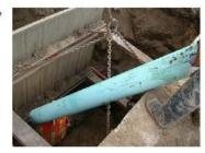
Lower the new pipe into the trench with a rope or any other safe method that will not endanger the labourers below.
