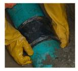
This type of coupler is used to connect pipe in a gravity flow system i.e. the sanitary sewer system.
