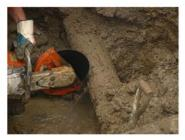
De-energize and/or remove water main if it is in the excavation and cannot be properly supported during the sewer main repair. Additional preventative measures and disinfection must be adhered to, to prevent contamination of the water main.
