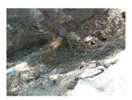
Cover services connection and mains with 150mm (6inch) of granular material and compact. Use spoil material if suitable. If not bring in clean backfill material.
