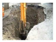
When excavating, watch the trench for any unmarked utilities. Note that the asphalt at this excavation has not been cut.
