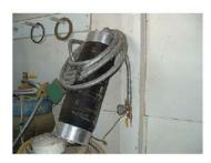
A sewer plug is installed in the sewer main, and the sewer pumped to the next available manhole to eliminate the flow of sewage at the repair.
