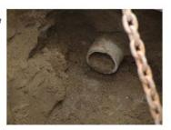
Expose and clean around both ends of failure, (inside and outside).
