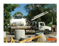
Vac-Truck is used to pump out and collect water and other liquid waste from the excavated area of damaged sewer line.
