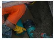
Align the replacement pipe and the existing pipe and tighten the 2 stainless steel clamps.
