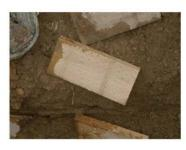
The treated wooden blocks are used to support pipes, clamps and coupler.
