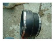
This type of coupler is used to connect pipe of different outside diameters.
