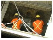
Measure between the ends of existing pipe and relay measurement to top labourer. It is beneficial to take measurements from the invert and top of pipe (pipe may not be square) to ensure that the new pipe is cut to the proper length.
