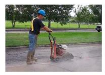
The Asphalt/Concrete saw is used to cut asphalt concrete.
