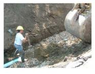
Place bedding over top of the pipe and compact. A walk behind tamper will be required for this process.
