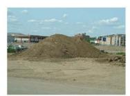
Backfill material should be free from loam [fertile material], sod, boulders or foreign material and frozen lumps.
