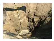
If soil conditions at base of excavation are unstable, remove unsuitable material and replace with crushed rock and/or granular material.
