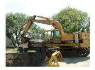
The excavator/backhoe is used to excavate but can also be used to lift heavy equipment like shoring into and from excavations.
