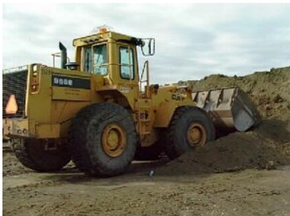
Figure 97 - Front End Loader
