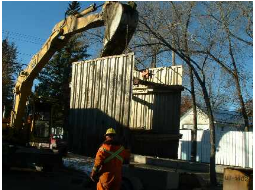
Figure 25 - Shoring on Trailer.
