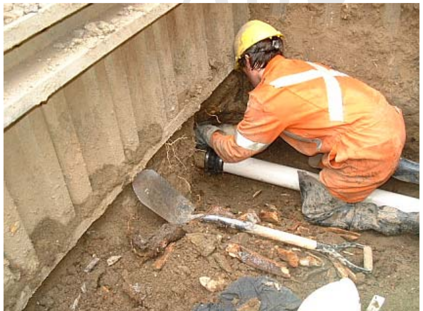
Figure 62 - Tighten Coupler
