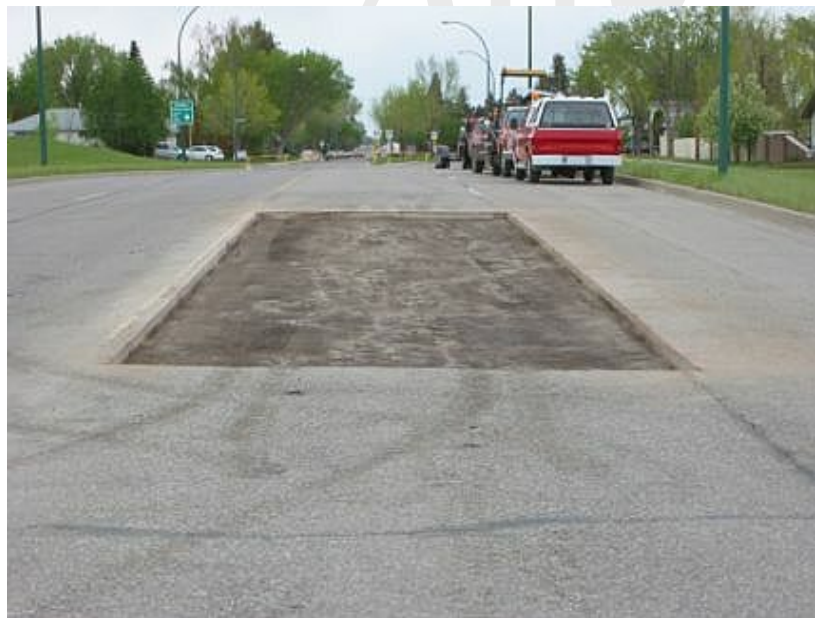
Figure 74 - Finished Backfill
