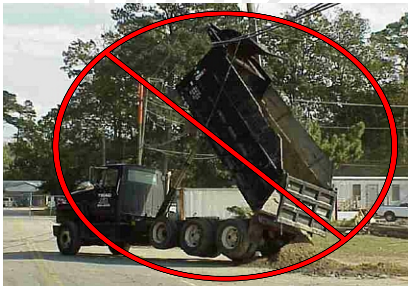
Figure 22 - Truck contacting overhead power lines.
