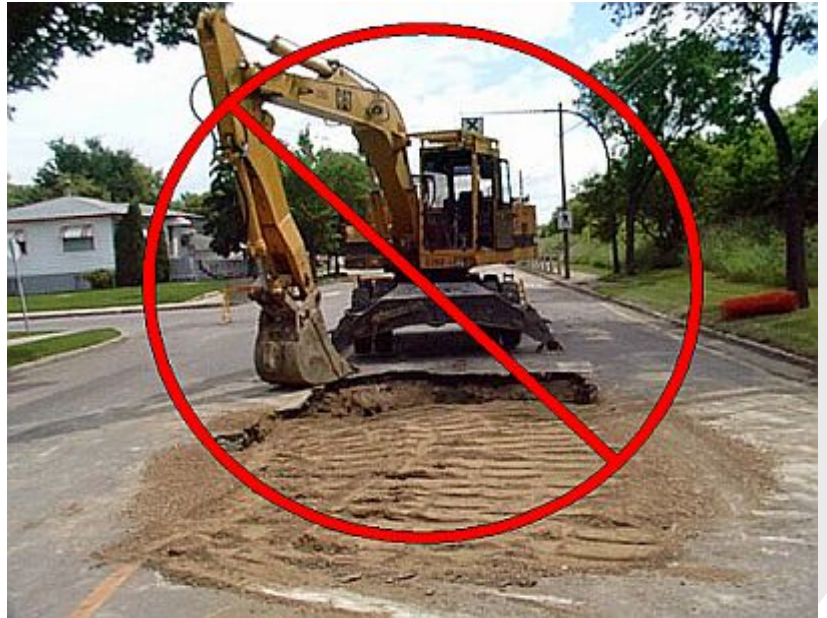
Figure 73 - Excavator/Backhoe backfilling
