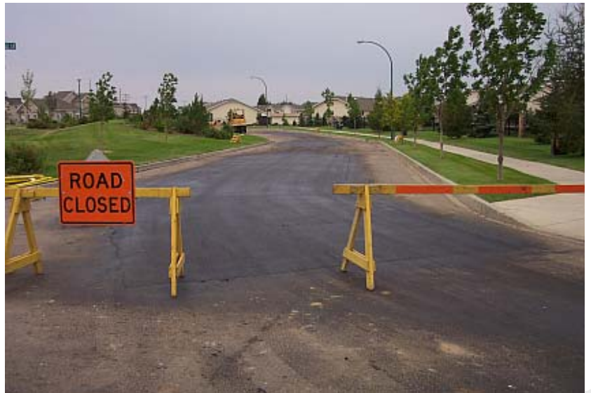
Figure 77 – Traffic Control Devices
