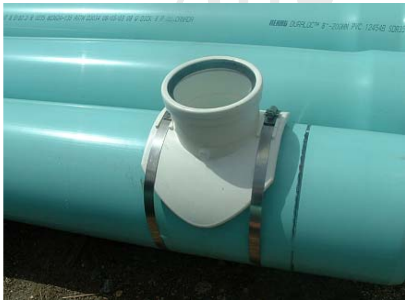
Figure 54 - Service Saddle Installed
