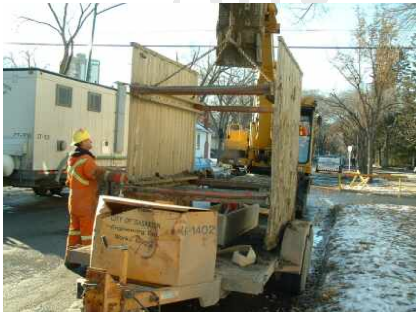
Figure 26 - Shoring being lifted off the trailer.
