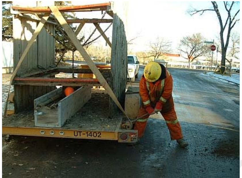
Figure 13 - Shoring on Trailer
