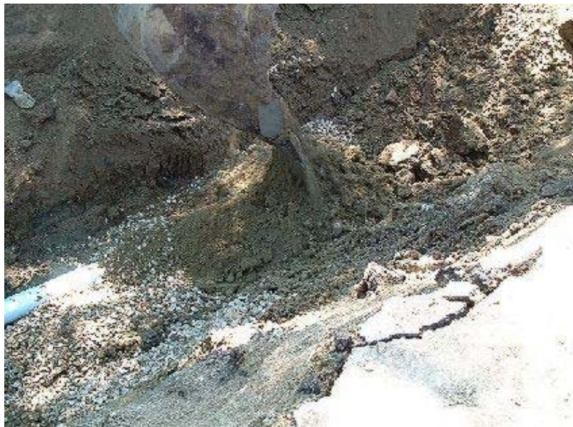
Figure 65 - Backfill
