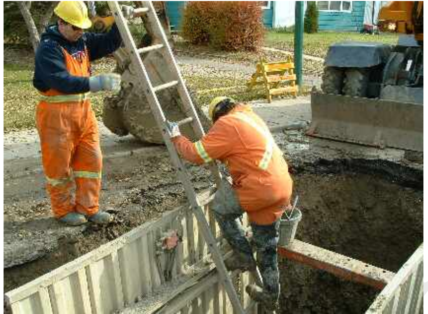
Figure 29 - Entering Excavation
