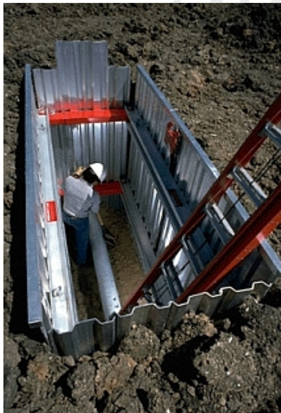
Figure 28 – Shoring with Endplates.
