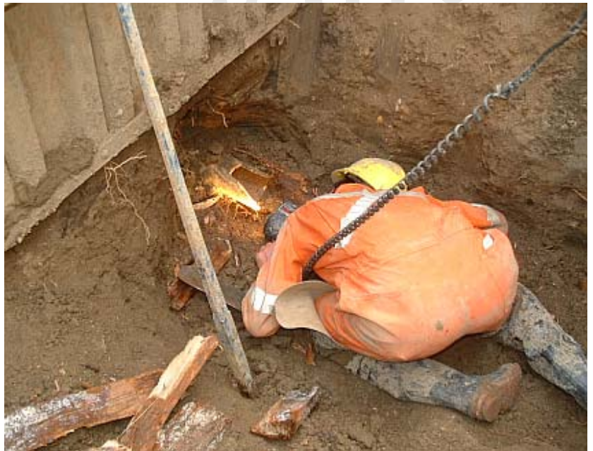
Figure 40 - Inspect Sewer Pipe
