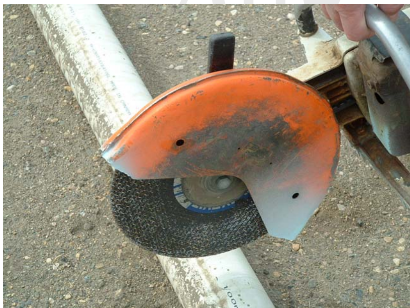
Figure 58 - Cutting Pipe
