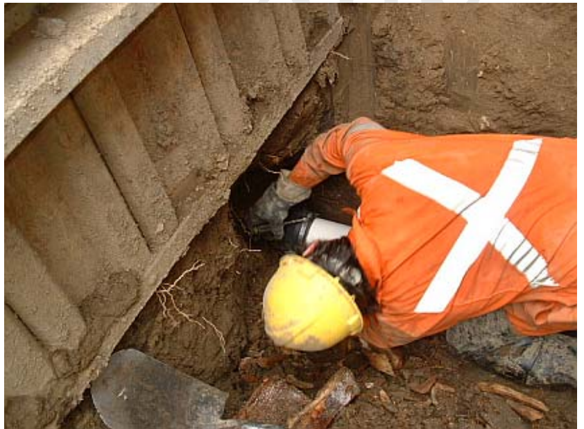
Figure 60 - Aligning the Coupler
