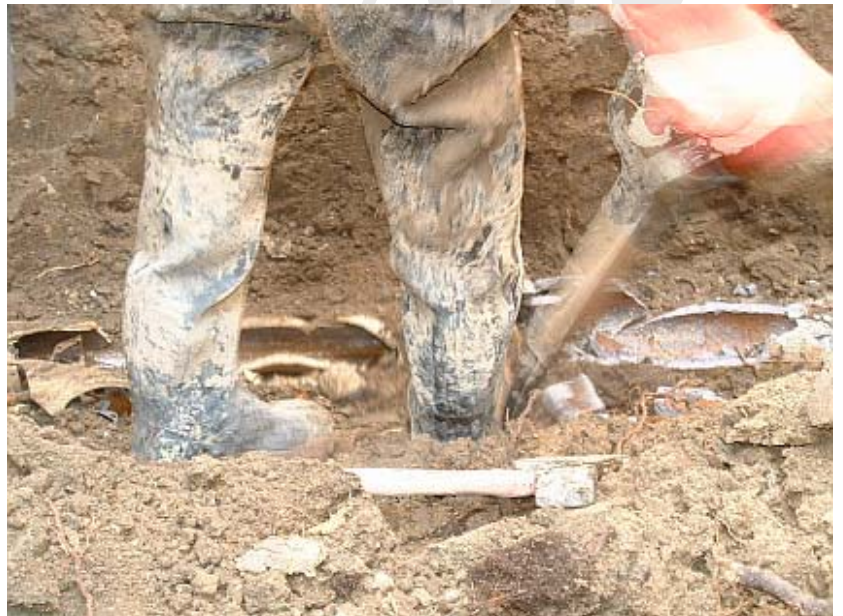
Figure 38 - Remove Pipe
