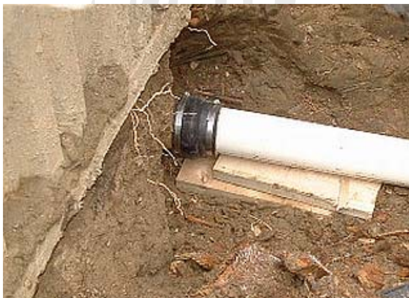
Figure 46 - Coupler Installed
