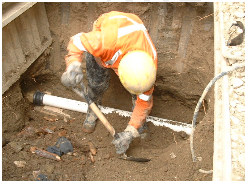
Figure 64 - Backfilling Sewer Connection
