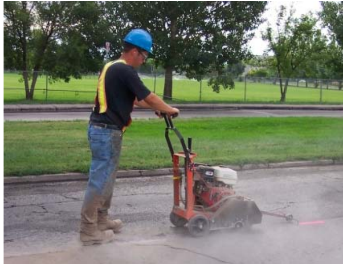
Figure 11 – Cutting Asphalt
