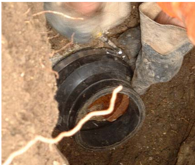
Figure 45 - Install Coupler
