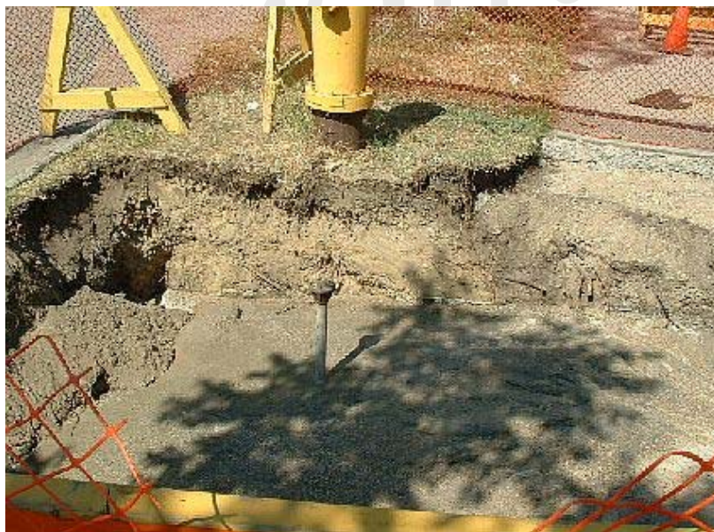
Figure 66 - Non-shrink backfill
