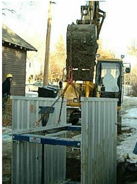
Figure 27 - Shoring Installation
