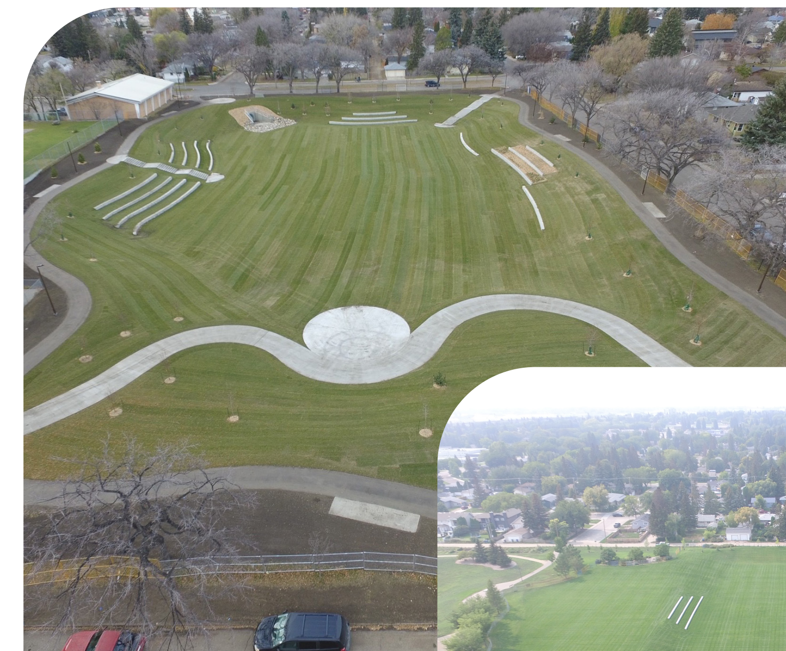
WW. Ashley Park Dry Storm Pond
