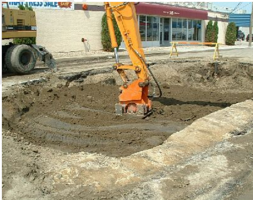
Figure 90 - Hydraulic Tamper
