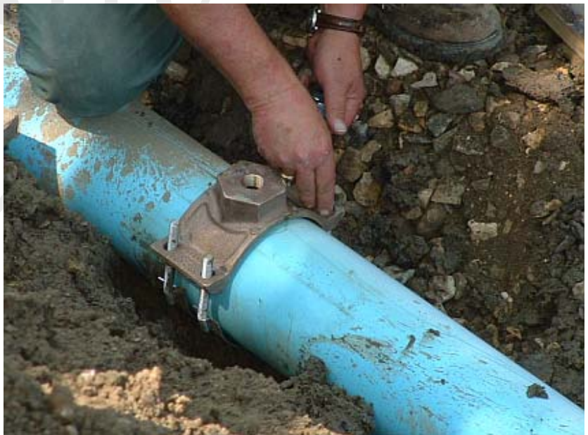
Figure 52 - Service Saddle Straps
