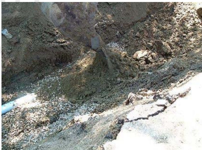
Figure 84 – Backfill
