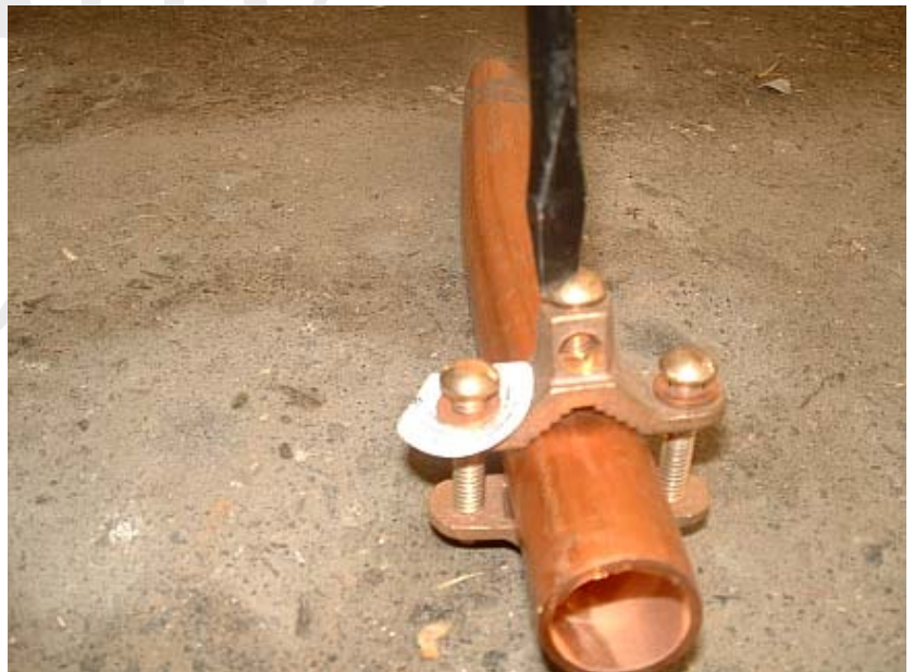
Figure 72 - Loosen Top Screw
