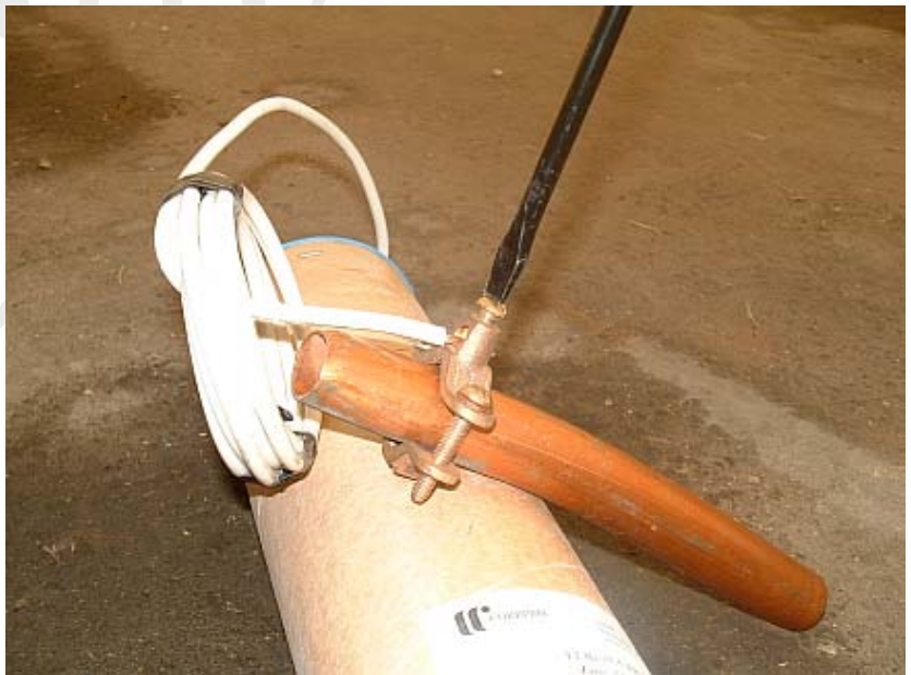
Figure 74 - Tighten top Screw
