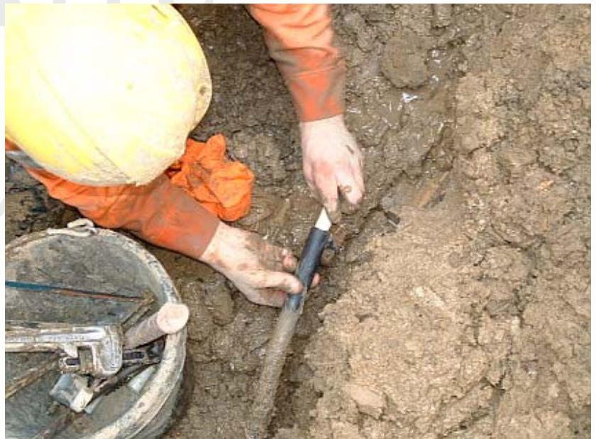
Figure 44 - Inserting the Insert
