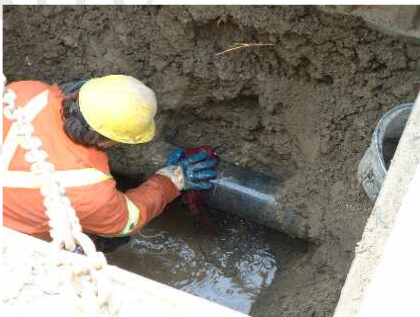
Figure 50 - Clean Section of Pipe
