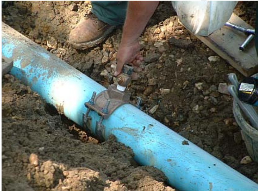
Figure 57 - Installing Main Stop
