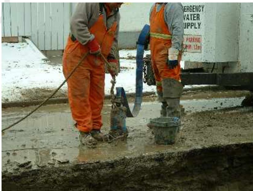
Figure 30 - Submersible Pump
