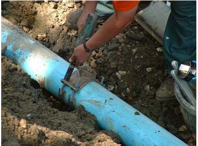
Figure 55 - Tighten With Drill
