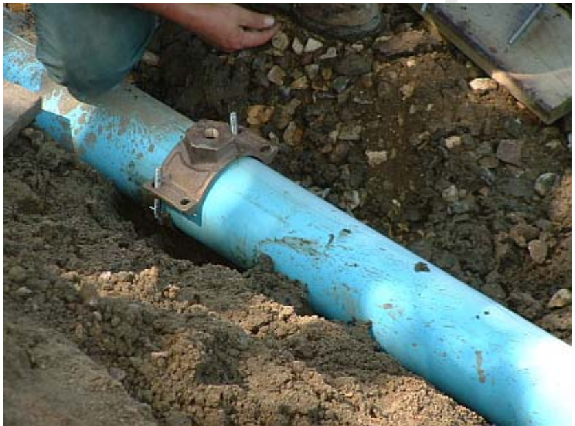
Figure 51 - Service Saddle Top
