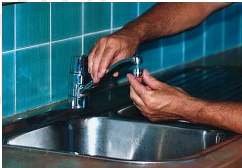
Figure 78 - Removing Tap Aerator
