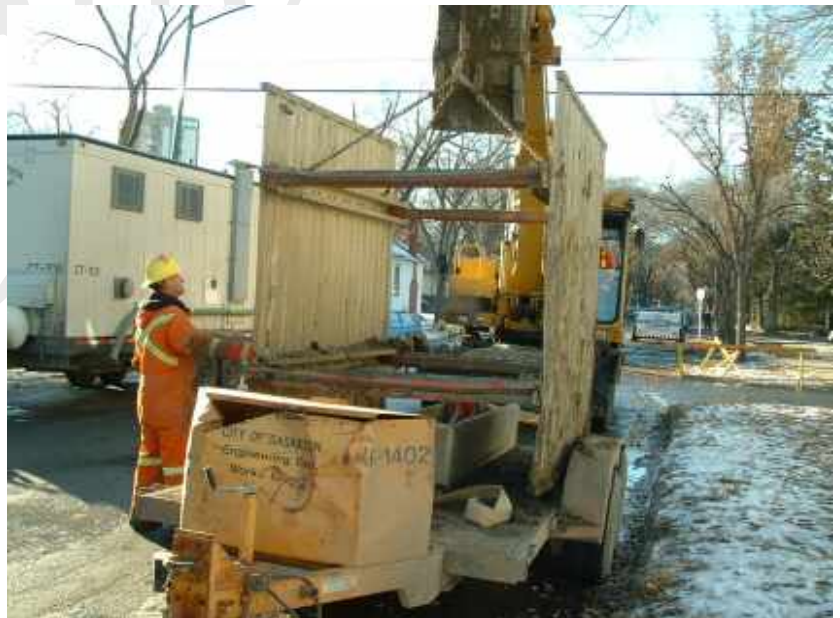
Figure 32 – Shoring Installation.
