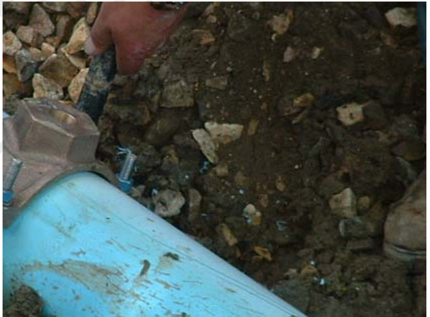
Figure 56 - Alternate Tightening Pattern
