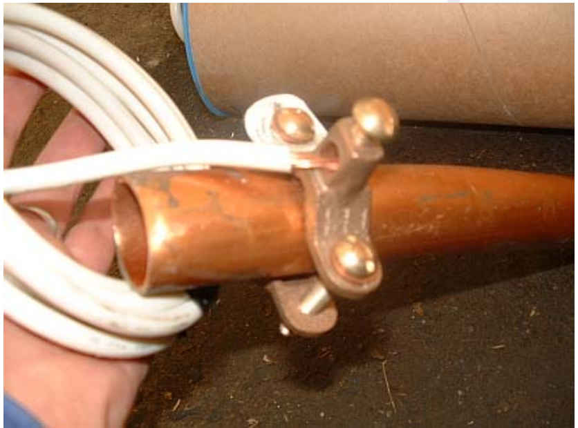
Figure 73 - Insert Anode Wire
