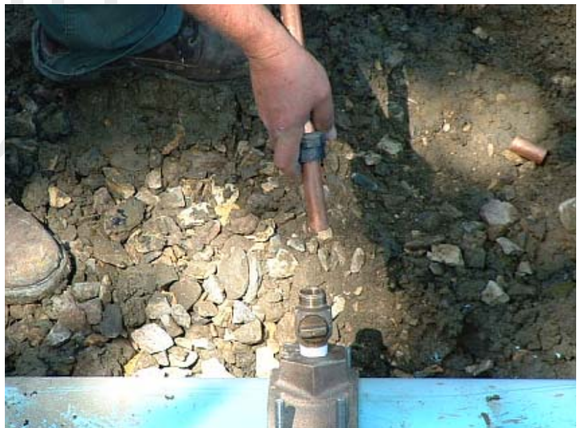
Figure 48 - Removing Pipe
