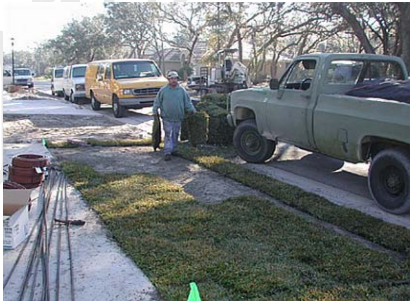
Figure 94 – Restoration of Water Connection
