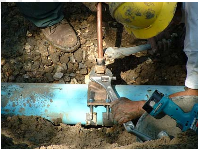
Figure 66 - Tighten the Main Stop
