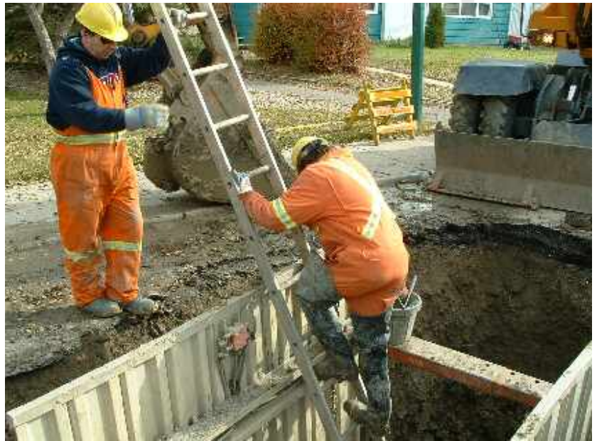
Figure 37 – Labourer Entering Excavation
