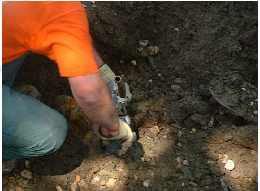
Figure 60 - Cut Pipe
