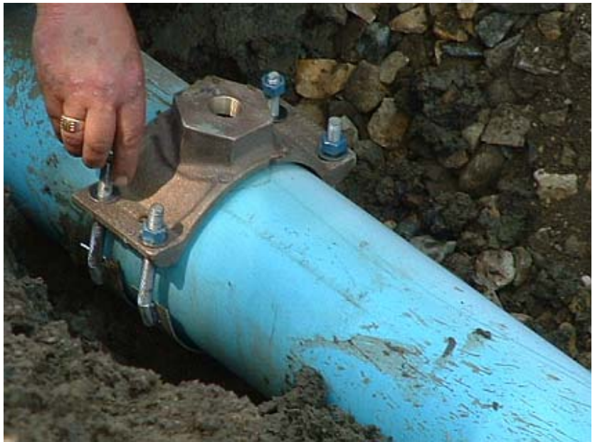
Figure 53 - Service Saddle Nuts
