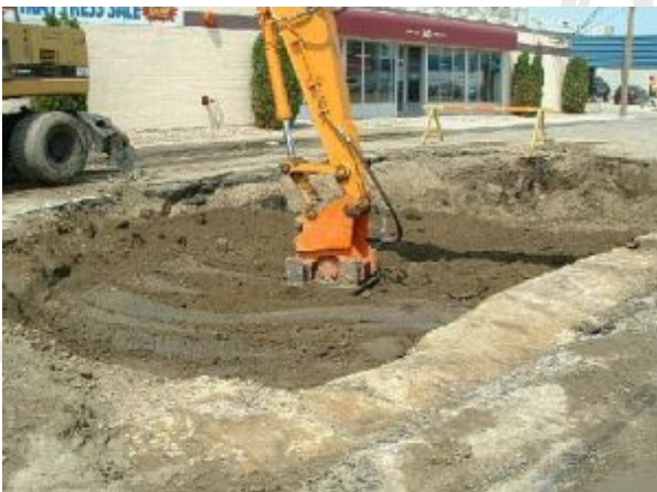
Figure 116 - Hydraulic Tamper [excavator attachment]
