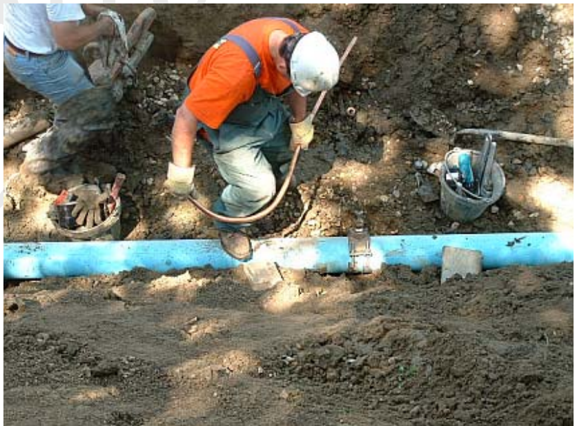
Figure 62 - Bending Pipe
