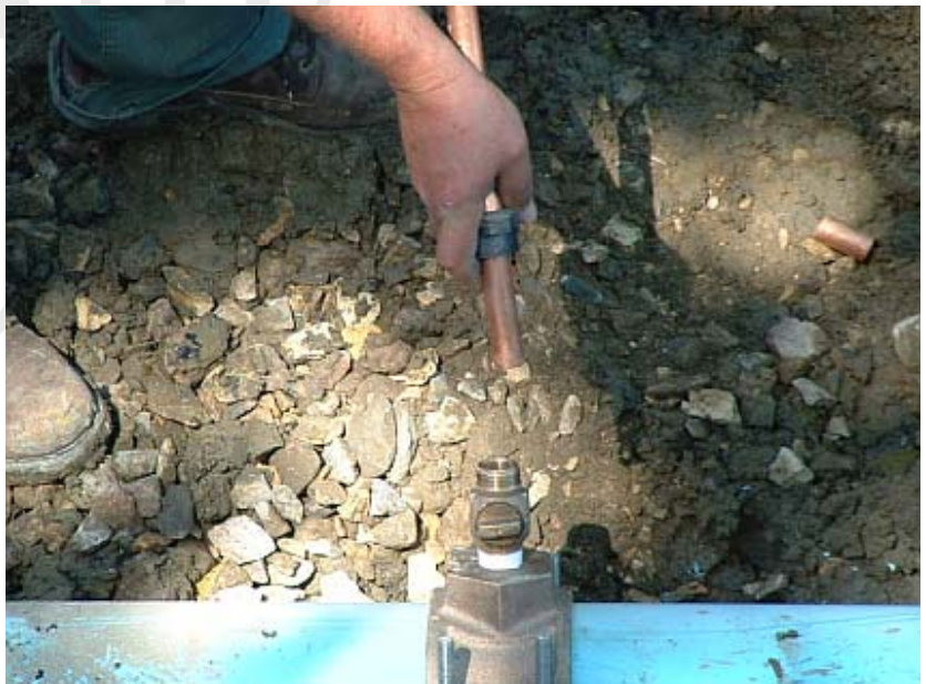
Figure 64 - Main Stop Connection
