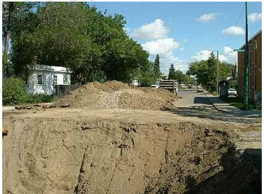
Figure 20 –Spoil Piles
