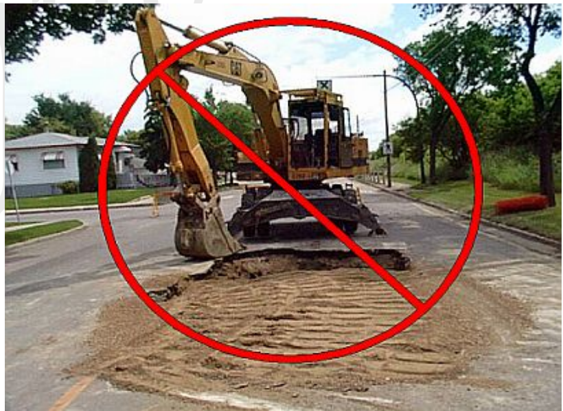
Figure 92 - Tamping with the Excavator/backhoe
