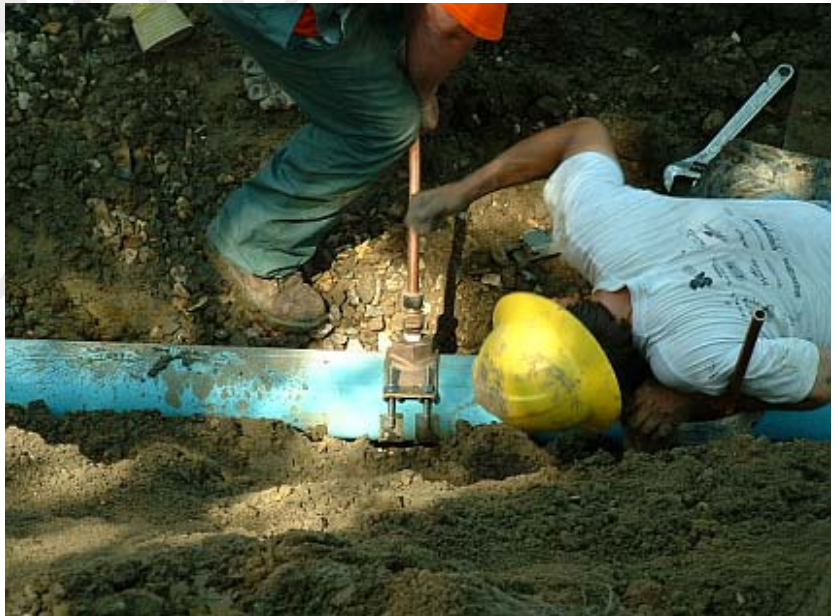
Figure 58 - Inserting Pipe into Main
