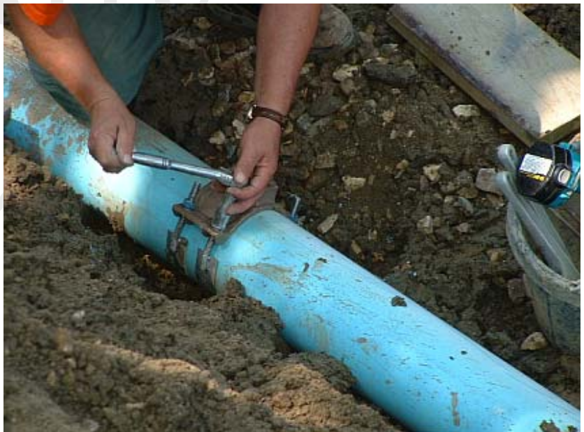
Figure 54 - Tighten With Strong Arm
