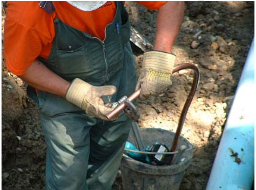
Figure 61 - Cutting Copper Pipe
