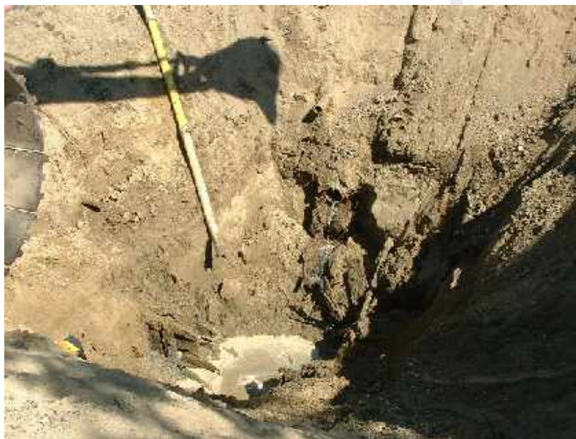
Figure 83 - Saturated Soil
