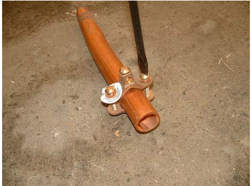
Figure 71 - Tighten Clamp onto Pipe
