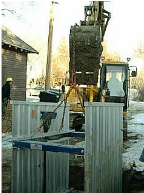
Figure 33 – Shoring in Excavation.
