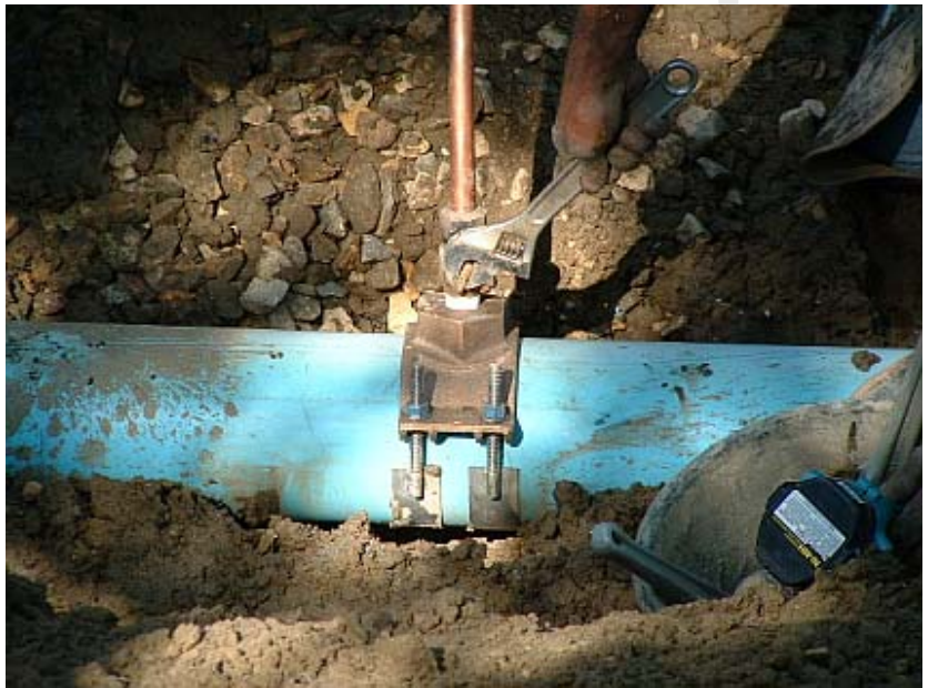
Figure 67 - Opening the Main Stop
