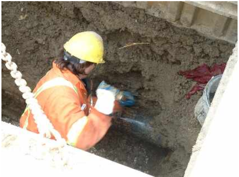
Figure 39 - Excavating with tunnelling shovel
