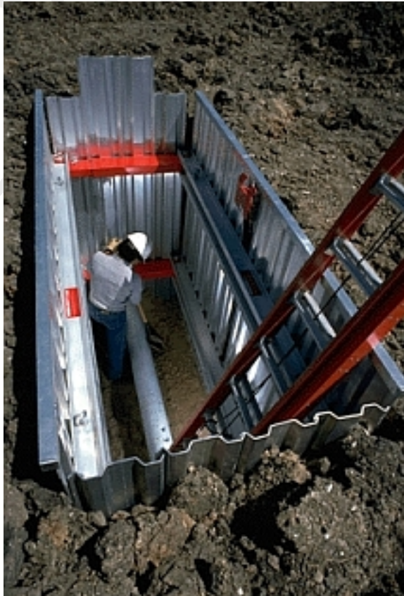
Figure 34 – Shoring with Endplates
