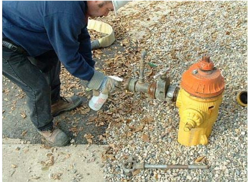
Figure 79 - Disinfecting Throttle Valve
