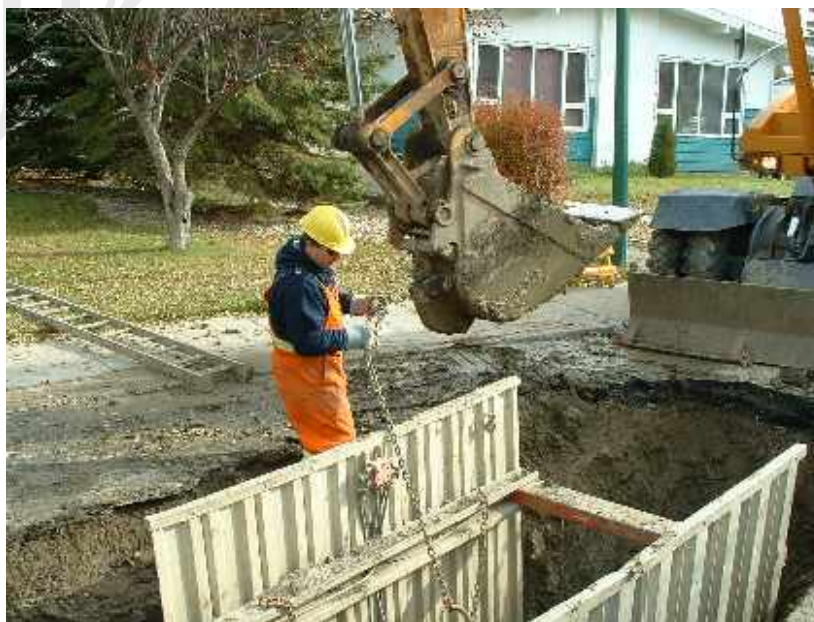
Figure 82 – Removal of shoring
