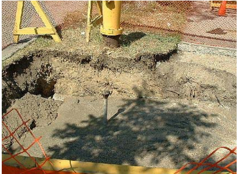
Figure 85 - Non-shrink backfill
