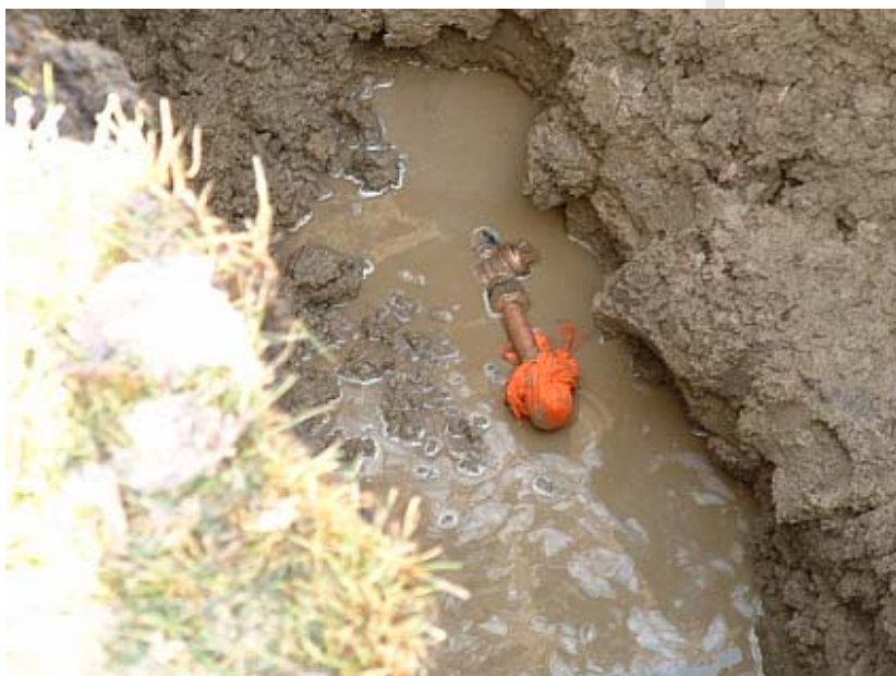
Figure 49 - Protect Pipe from Debris
