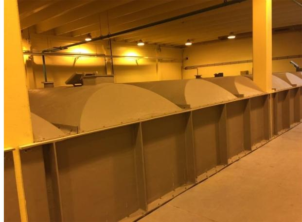
The above pictures show the WWTP Dissolved Air Flotation (DAF) tanks before and after covers have been added to reduce odour. The thickening process allows more solids to be removed from wastewater and contributes to the clarification process.
