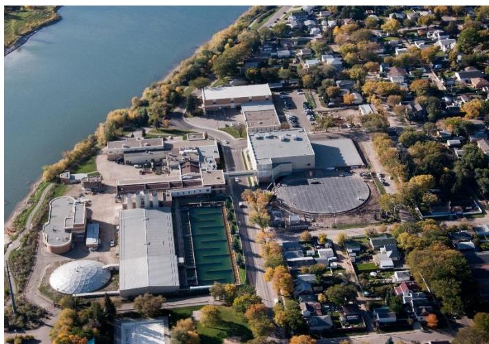
**The Water Treatment Plant** (WTP) supplies all consumers with safe and reliable, high-quality drinking water. Core functions include operating and maintaining the South Saskatchewan River Raw Water Intake, the WTP, and three potable water storage reservoirs with a capacity of 114 million litres.
