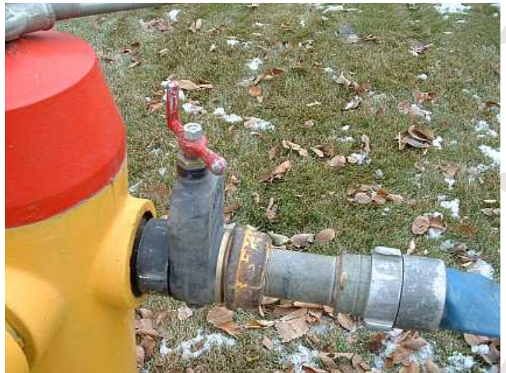
Figure 55 - Hydrant Valve and Hose
