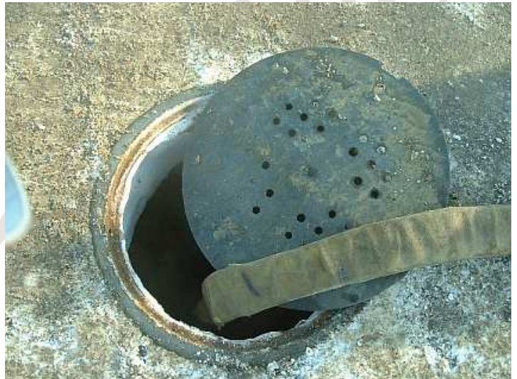
Figure 56 - Hydrant Hose in Manhole
