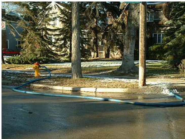
Figure 7 - Flushing
