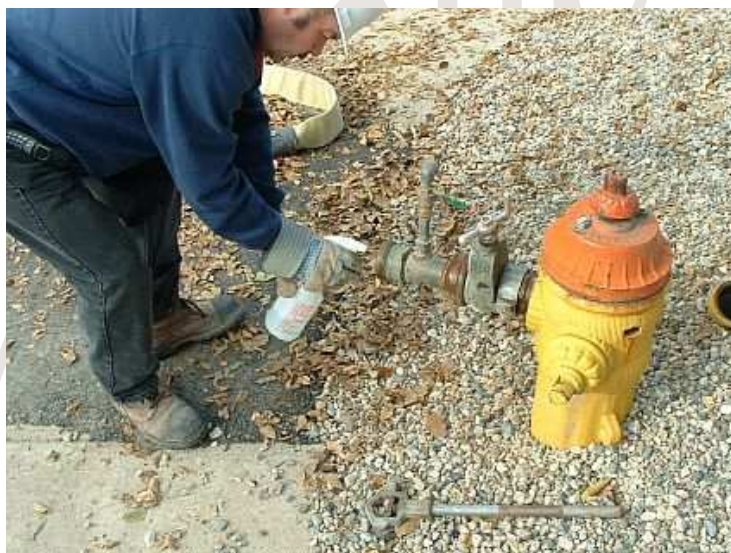
Figure 4 - Disinfect gate-ball valve
