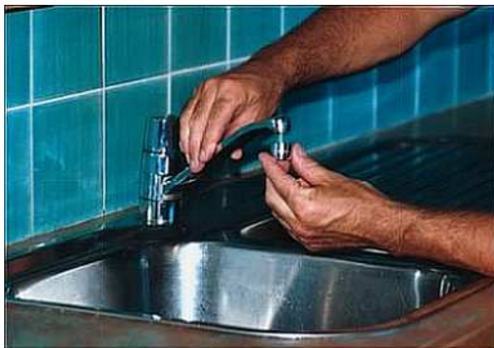
Figure 9 - Removing Tap Aerator
