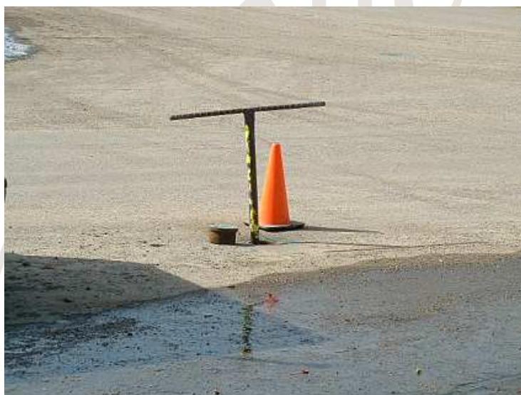
Figure 6 – Opening a Valve
