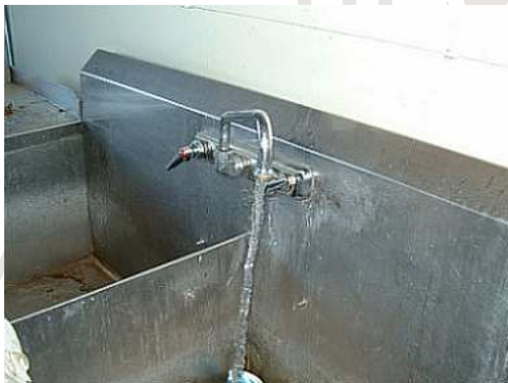
Figure 10 - Flushing Through a Tap
