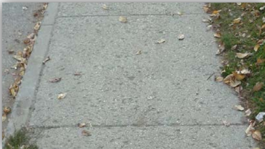
Light Severity – No Treatment
