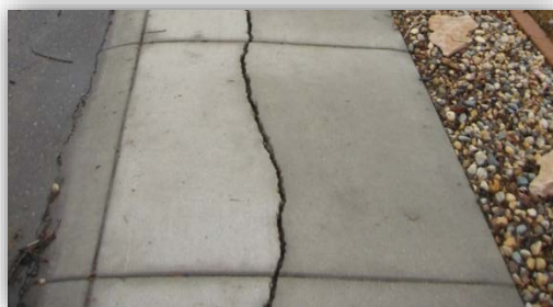
Repair - Crack Fill
