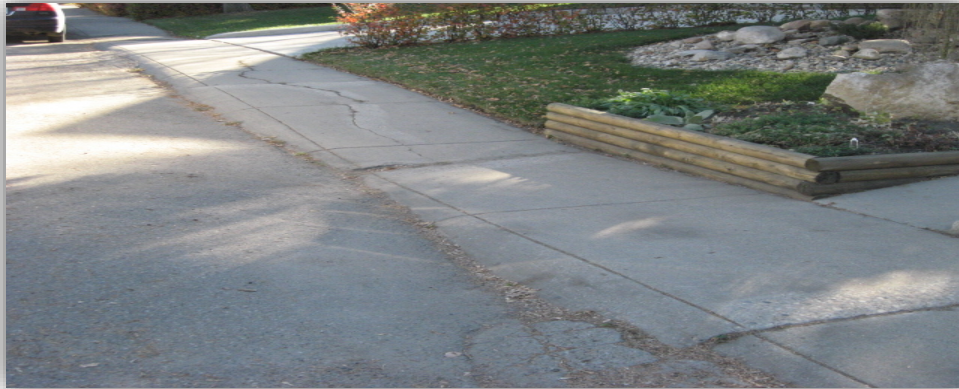
Utility Settlement – Mud Jack or Replacement
