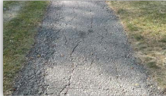
Fair Condition Asphalt Overlay - Replacement
