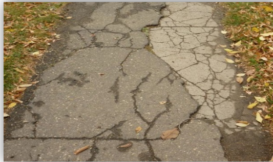
Poor Condition Asphalt Overlay - Replacement
