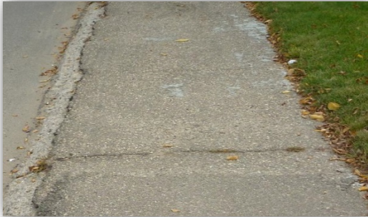
Good Condition Asphalt Overlay Curb Deteriorated - Replacement
