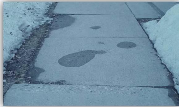
Mud Jacking or Replacement
