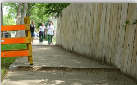
Repair – Grinding or Saw Cut
