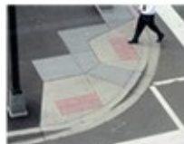
Addition of curb ramps at intersections to enhance accessibility
