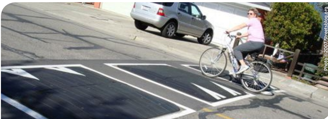
Figure 5.13 Speed cushion example on Bayview Drive in Alameda, CA
