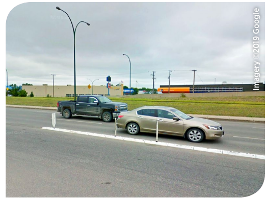
Figure 5.19 - Intersection channelization at 22nd Street and Fairmont Drive
