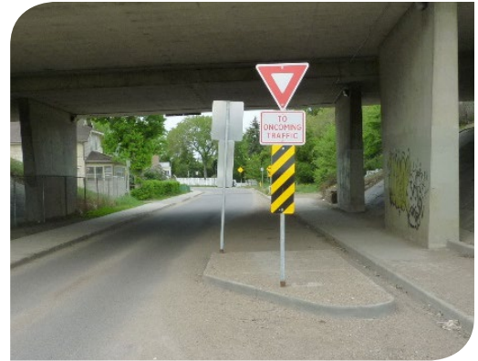
Figure 5.6 - Pinch Point on Saskatchewan Crescent (Nutana Neighbourhood) indicating that traffic must yield to oncoming traffic.
