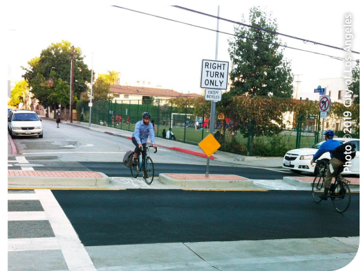
Figure 5.20 - Raised median through intersection
