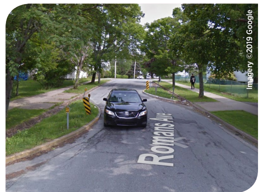
Figure 5.8 - Chicane on Romans Avenue in Halifax, NS
