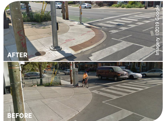
Figure 5.7 - Corner Radius Reduction on Davenport Rd. and Christie St. in Toronto, ON
