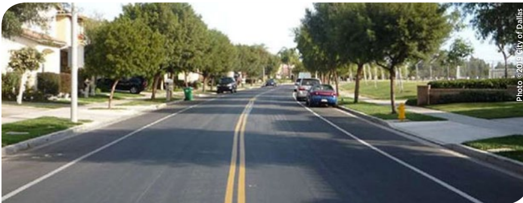
Figure 5.10 Lane narrowing using pavement markings
