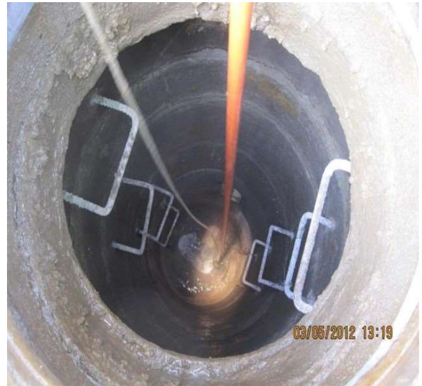
Closed Circuit Television Work
