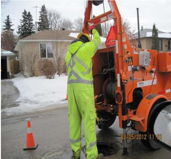
Closed Circuit Television Work
