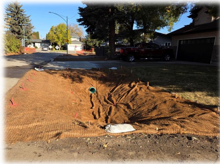
Figure 7: Ditch Improvements Under Construction in Montgomery Place
