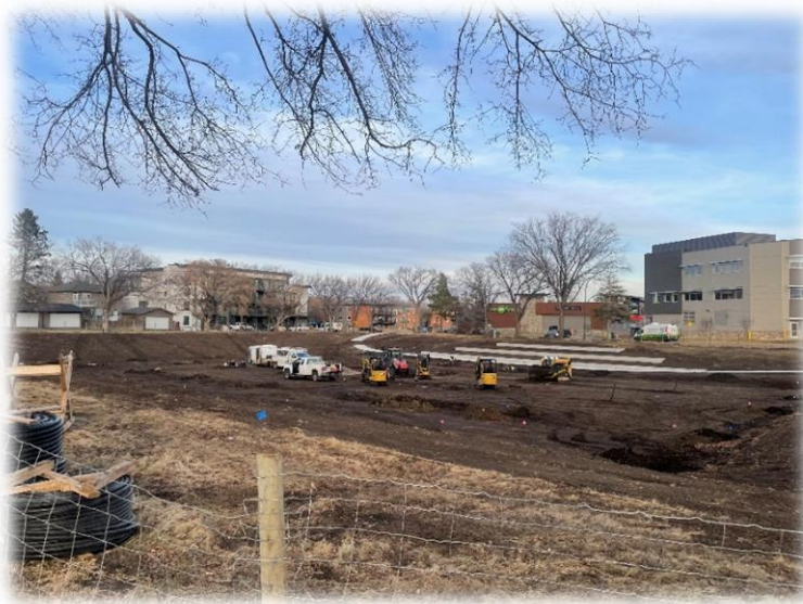
Figure 3: Cumberland Park Landscape Construction
