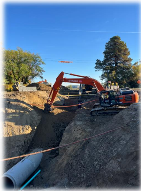
Figure 4: USask Dry Pond Storm Sewer Construction
